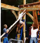
Builder and musician Will Anderson (far left) uses an A-1 of help from the friends to raise a section of his new barn's timber frame. See "Out of the Woods," page 104. By JOE CARRAS
