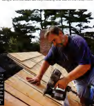
Double-thick lead-coated copper protects every corner that water flows down, so it's not a matter of if, but when it rains, the roof will hold.
