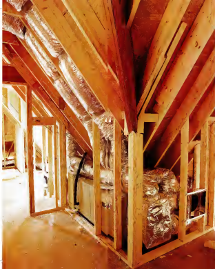
Right: Johnson's duct (top) carries air to and from the basement furnace. Wire-reinforced flexible plastic ducts carry the same purpose for a 25-ton electric heat pump installed behind a base wall on the second floor (left). A number of HVAC contractors Ron Jones came for the aid of a flexible ducts on a run on the second floor (center).
