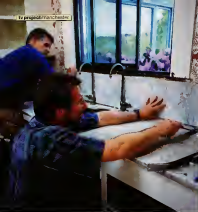
Before Tom takes the demolition crew into the walls, he removes any fixtures and anything worth saving. In the old master's pantry, Tom and T.O.H. master carpenter Steve Adams are prying him to carefully dismantle an antique marble counter with a copper sink, which they hope to reuse somewhere else in the house. (Left) Tom gently pushes away the second floor ceiling so that he can replace it when he has finished constructing the new walls. The 19th-century moldings have survived two previous renovations.
