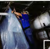
A member of the Dec-Ten crew begins to peel the area around the asbestos-encapsulated water tank and boiler by taping up 6-mil plastic to the ceiling joists (above). With the material fully encapsulated in a wet (below), removal can begin. The enclosed, lower asbestos area under tank prevents air from getting around or outside (right).
