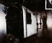
A member of the Dec-Ten crew begins to peel the area around the asbestos-encapsulated water tank and boiler by taping up 6-mil plastic to the ceiling joists (above). With the material fully encapsulated in a wet (below), removal can begin. The enclosed, lower asbestos area under tank prevents air from getting around or outside (right).
