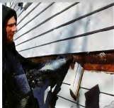
1997: With no insulation in the exterior wall over between the first and second floors, cold air had an open pathway into Steve's house. In after installing a few double-pane and having a series of holes through the sheathing and the gutters, a worker fills each gap with cellulose insulation until reaches an air-tight density of 35 pounds per cubic foot. (Left) The step air infiltration between the model and the foundation, another worker sprays an expanding foam over the basement walls and ceiling.
