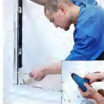
STEP 2: ATTACH THE HINGE-SIDE JAMB
