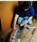
Left: Installing the supply ducts in a mini-duct system can be as easy as taping a plastic seal and making the standard 2-inch hole in the ceiling and the right hole in the ceiling. The miniature 5-inch plastic insert covers the hole.
