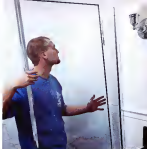
STEP 4: INSTALL THE REMAINING SIDE JAMB
