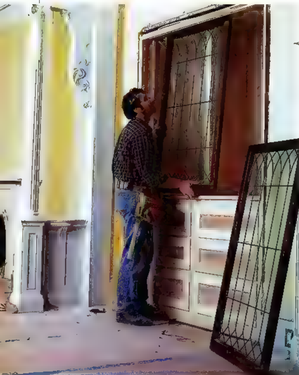
ABOVE Norm Abram fits old leaded-glass doors from the original china cabinet on the first floor into a matching cabinet he crafted for the Beliveaus' dining room on the second floor. The doors slide smoothly on tracked wheels, while the cabinet's six dovetailed drawers glide in and out on full-extension slides hidden on the drawers' undersides. Norm surrounded the new cabinet with a mitered casing (RIGHT), custom-milled to match the two-part molding profiles Tom Silva installed in the rest of the house.
