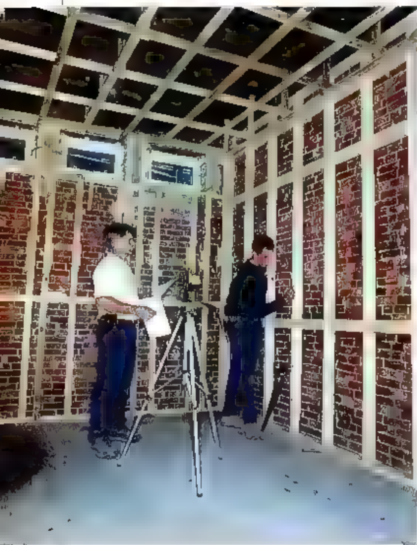
After gutting the old second-floor kitchen, bath, and back staircase, Tom furred out the walls and leveled the ceiling to get a kitchen with the biggest possible footprint. ABOVE: Using a laser level, Tom and electrical contractor Allen Gallant decide where to rough in the kitchen’s wiring. RIGHT: Tom shims and screws a base cabinet to fit tightly against the wall.
