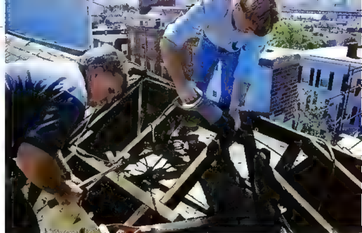
ABOVE: While tearing off the old roof, Tom Silva's crew and host Steve Thomas exposed the remnants of a small window's walk, where some long-ago owner once enjoyed the panoramic views. Tom surmises that the walk was covered over because it leaked so much, but its existence proves that a rooftop aerie was part of the house's original design scheme, not just a modern indulgence. BELOW: Dick Silva cuts the stringers for the stairway leading to the newly sheathed deck. The bird's-eye view (from the side of the house) shows how Tom sliced off the roof's peak to build the platform.
