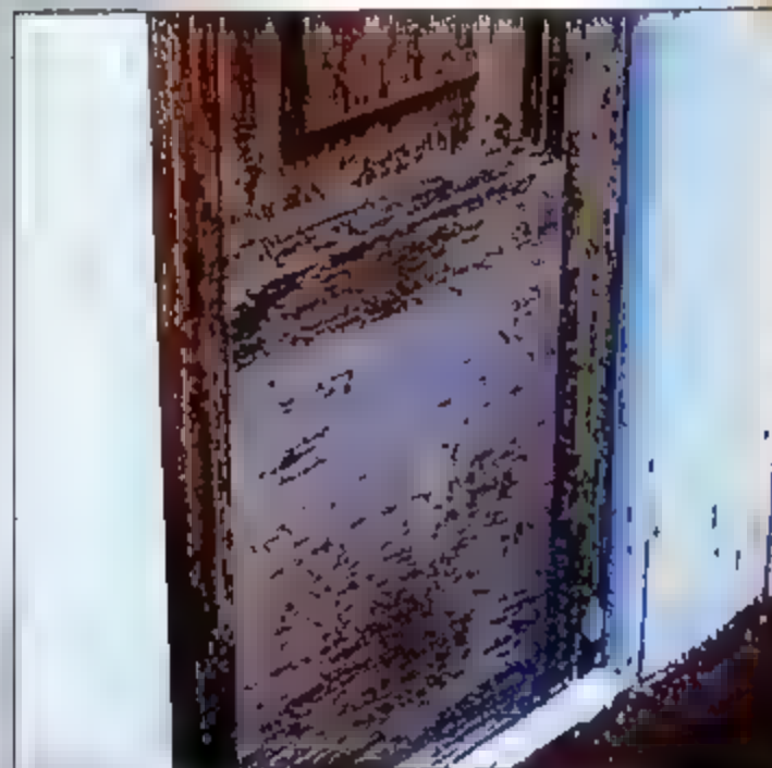
The toughest job for a clear finish isn't keeping out water; it's preventing the sun from breaking down surface fibers, as it has done on this varnished wood panel in Washington.
