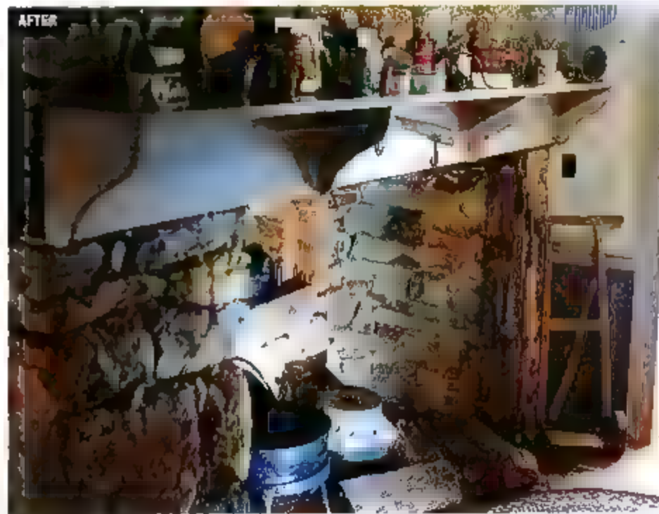
A cavernous early-19th-century cooking hearth, big enough to fit several boiling pots over the fire, suffered a sad fate for many decades, having been covered over and fitted with cabinets by previous owners (ABOVE). After tearing away bricks, plaster, and wood, the Nolls restored the 7-foot-wide fireplace, delighted to find within its limestone walls an original beehive oven (LEFT).
