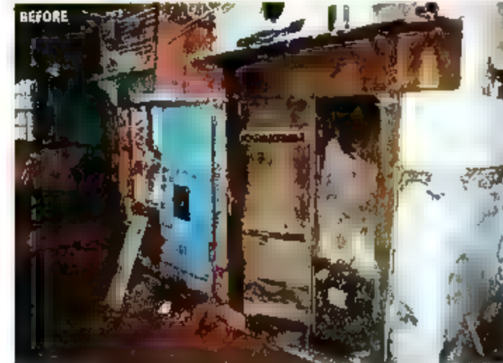
A cavernous early-19th-century cooking hearth, big enough to fit several boiling pots over the fire, suffered a sad fate for many decades, having been covered over and fitted with cabinets by previous owners (ABOVE). After tearing away bricks, plaster, and wood, the Nolls restored the 7-foot-wide fireplace, delighted to find within its limestone walls an original beehive oven (LEFT).
