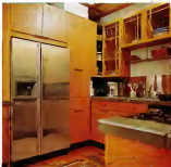
The backs of the upper cabinets (above) were glassed in to bring light in from the study across the hall. The stainless steel backsplash (left) goes to the ceiling, and the backsplash (right) goes to the ceiling.
