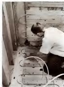
For his own remodelled bathroom in Zurich, Switzerland, plumber Dieter Freudenstein chose to warm the floor and walls. In 2007, he used a rubber mat to protect the PEX tubing and prefabricated panels. Further, he also installed a 6-gallon electric water heater (150,000 Btu) that keeps the water circulating at 80 degrees and supplements the forced-air heat.
