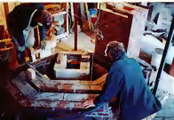
ABOVE: Building the stove requires careful planning because everything is assembled from the ground up. Alex, Alvin Barden, left, and an apprentice lay concrete floor joists onto which he built a warm bench wrapping around the perimeter of the stove. (LEFT) The 18-by-24-inch fluebox, back of heat-resistant brick and concrete, is designed for just a few logs at a time.
