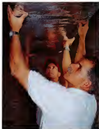
TO-H contractor Sam Selva helps Don fit a section of 24-inch-wide ductwork into the main basement trunk line. Don faced additional obstacles some of the framing sheet metal technicians that offers some options. A flexible collar on the plenum, where the ductwork connects to the furnace, effectively prevents noise from reverberating through the house.
