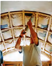
ABOVE: Using a gypsum flexible into a curved ceiling post and of 5-inch drywall. All from parts of these extruded ends by side with construction adhesive and screws to create 2-by-6-inch framing. Spacing construction adhesive into the joint, fill some carpenters in the case of the shingles and helps the drywall attached more securely than nailing alone. In some cases, using adhesive can also reduce the number of drywall features needed.
