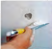
arrow. With a dollop of joint compound and a putty knife, Bob Thompson fills the dent created by a screw that has rusted from the stud. NOTE: Longer holes need something for the compound to adhere to, so Thompson applies a small piece of mesh before spreading on the compound.
