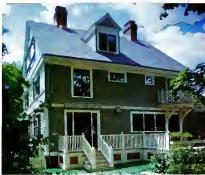
To the left, new position next to the kitchen, the door has access to the deck and backyard. A built-in bench doubles as a great bed, says Brooks. The back of the house is much more useful now than it has a wide deck and steps leading to the yard. A bike shed and off-street parking (to the right of the photograph, off the kitchen and driveway) are new features in this neighborhood.
