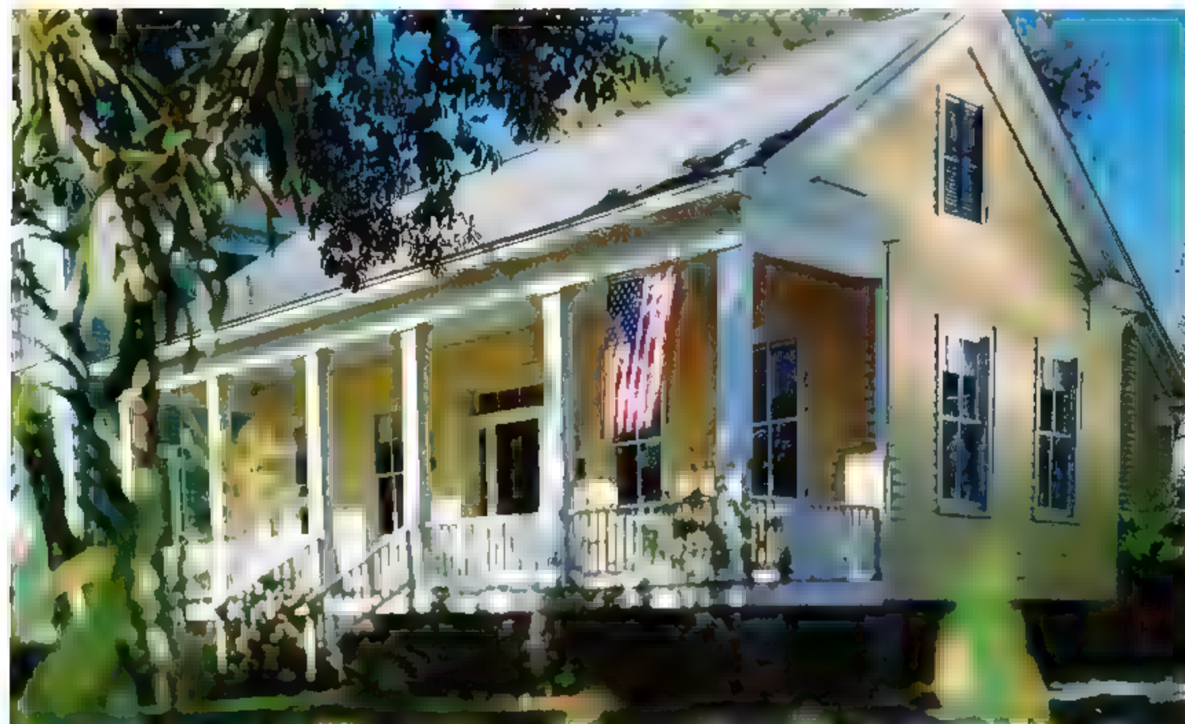
"Yellow Rose of Texas," p. 116. Vintage photos helped identify the style and location of former trim on this Greek Revival home in Texas.
