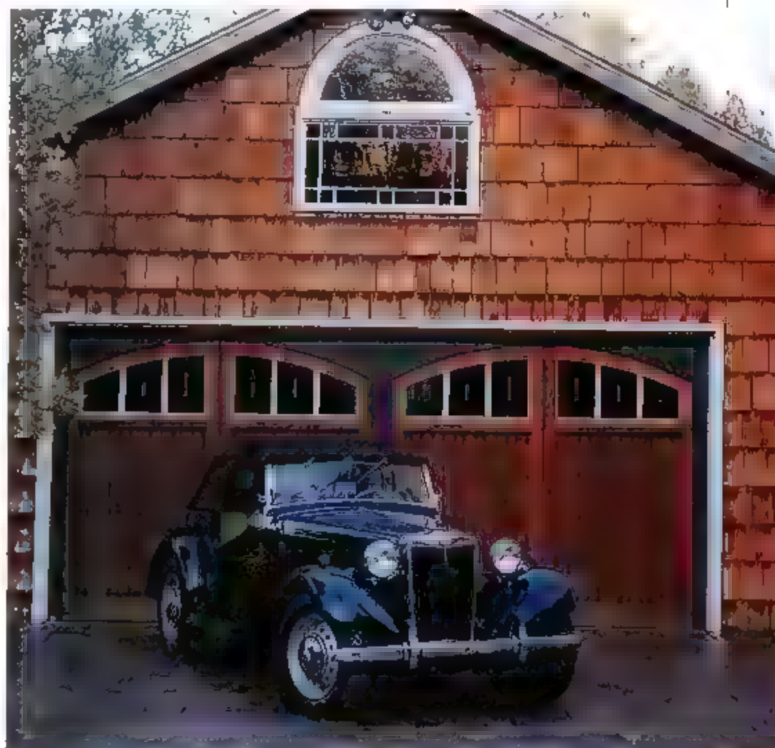
How many doors are in this garage? Though it looks like it has two out-swinging doors, it actually has just one overhead unit, made with stained cedar, painted trim, and curved windows.
