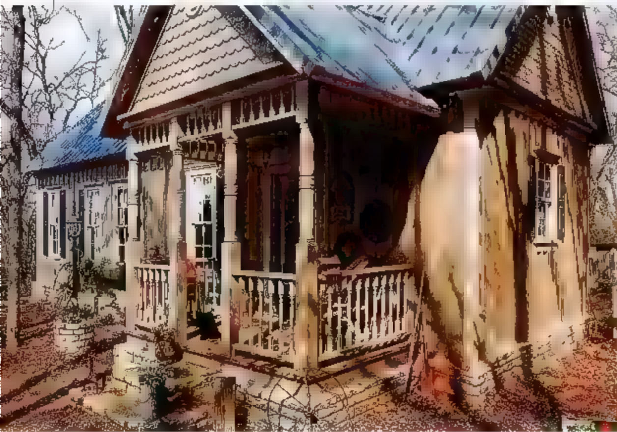
A new portico graces the entrance of Helen Kerwin's restored cabin (ABOVE) with cedar fish-scale shingles and a 12-over-12 roof pitch to match the original gable ends. BELOW: the abandoned house, ready for the move.
