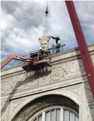
Shea's Performing Arts Center , Buffalo, NY Façade Restoration: January, 2004
