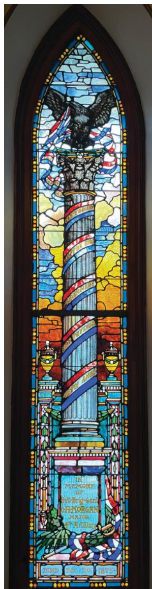
Above left, at the Cuban Embassy in Washington, D.C., Lynchburg Stained Glass removed the 1917 building's stained-glass skylight that crowns its four-story atrium, preserved it, re-leaded it, and reinstalled it. Right, Lynchburg Stained Glass removed, restored, and preserved eight historic stained-glass windows at the Chapel of the Centurion at the Fort Monroe National Monument in Hampton, Virginia.
