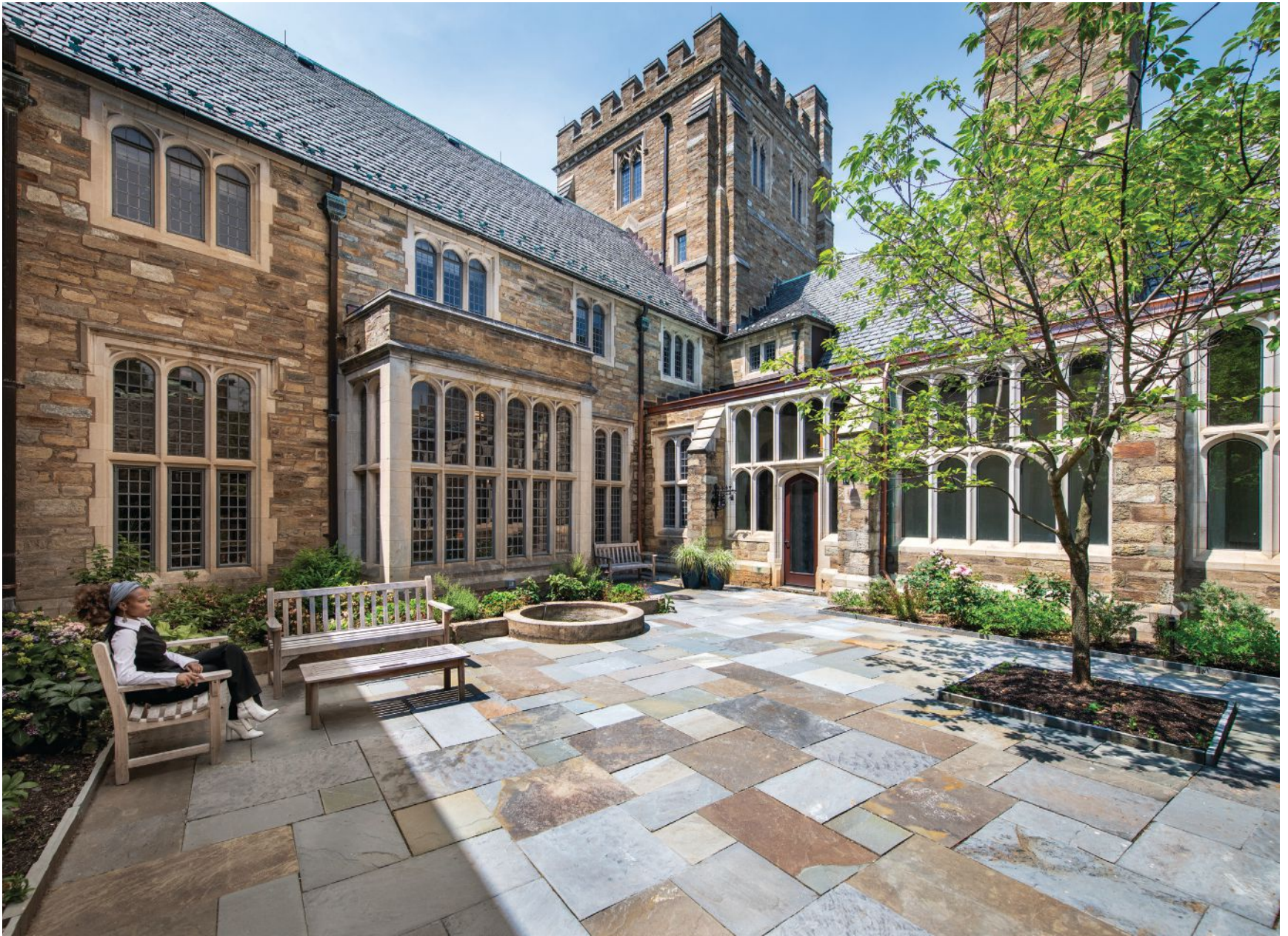
Above, an outdoor courtyard known as Garth, provides outdoor space within the building’s network of spaces. Right, the structure was pared back to the building’s foundations and exterior stone walls.
