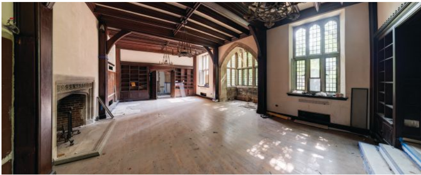
Top, the library after restoration and renovation, and above, before.
