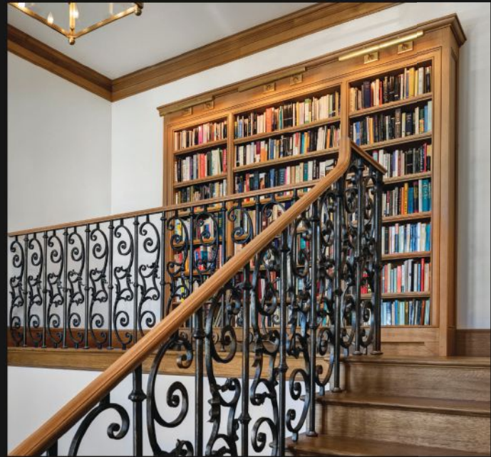
FORGED IRON BALUSTRADE. YALE UNIVERSITY. Robert A.M. Stern Architects. Dimeo Construction.
