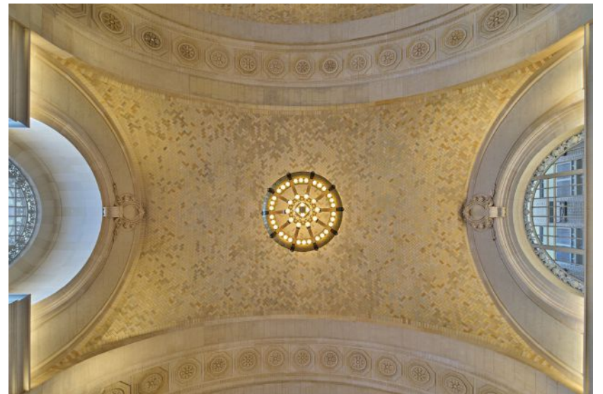
The Guastavino tile-vaulted ceiling in the historic waiting room. Before: Photo by James Haefner , After: Photo by Jason Keen
