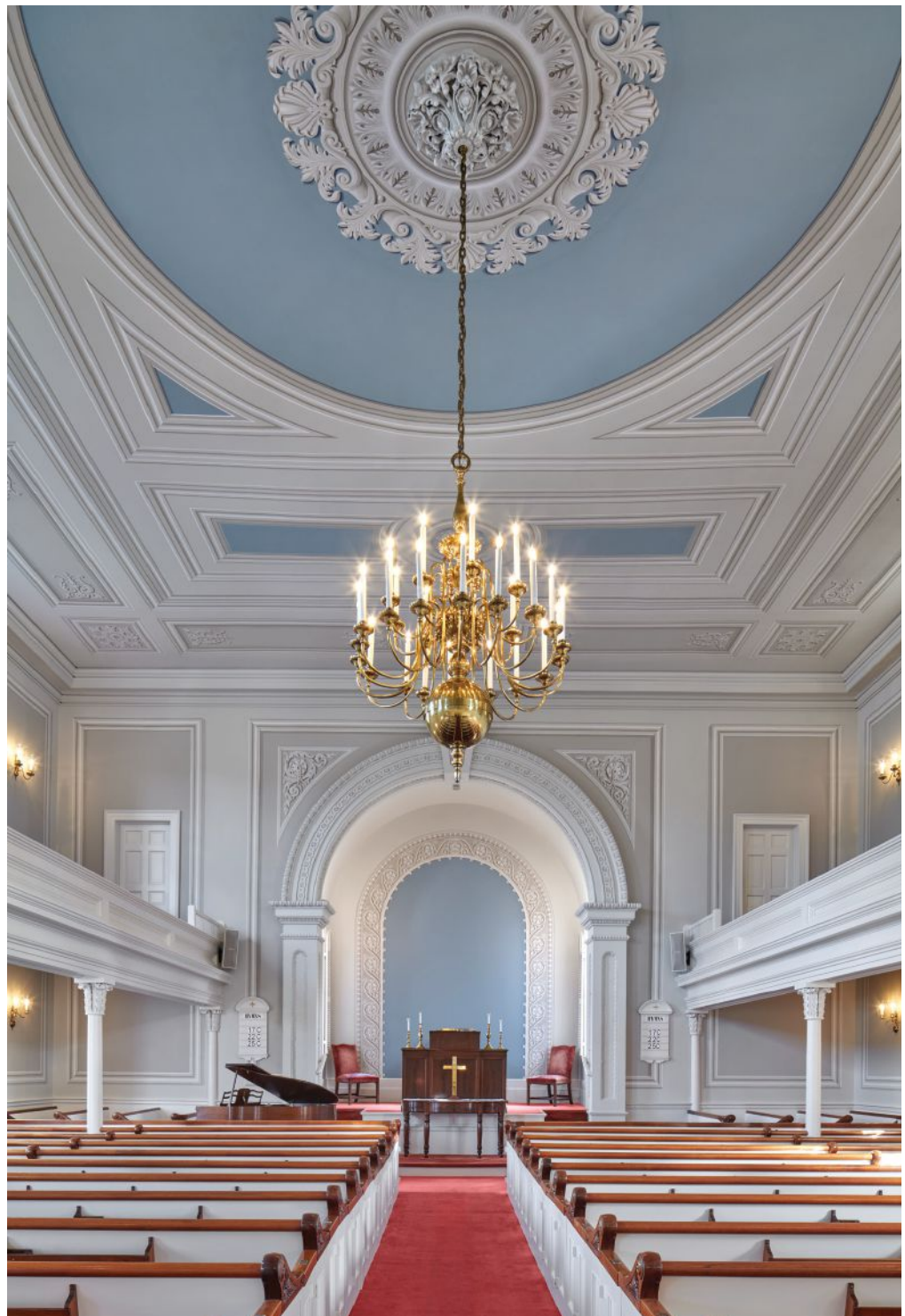
Overall view of First Church of Christ after the completion of the work. Photo by Robert Benson Photography
