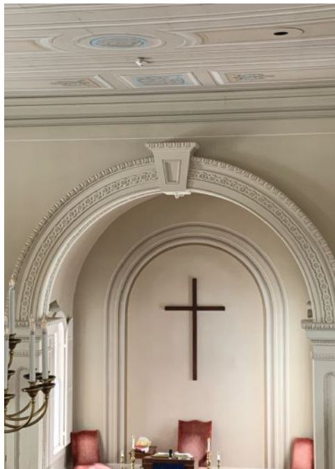
The altar arch, before and after. A detail of the completed trompe-l'oeil arch border on the church wall.
