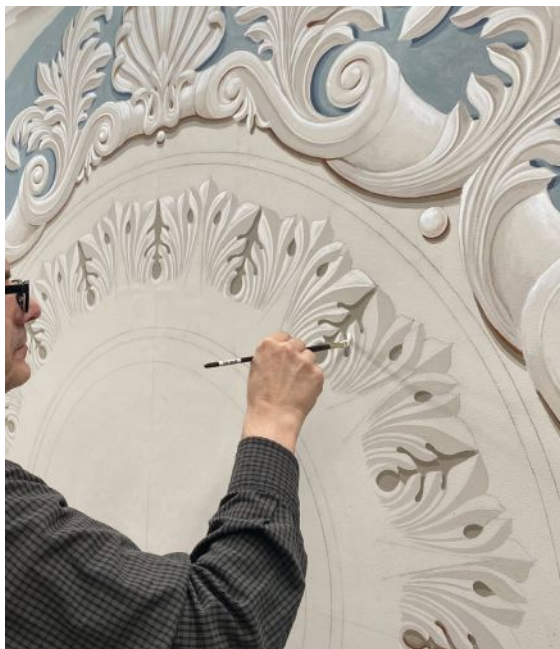
A John Canning & Co. artist works on the ceiling's trompe-l'oeil rosette of scrolling leaves. Right, the ceiling medallion.
