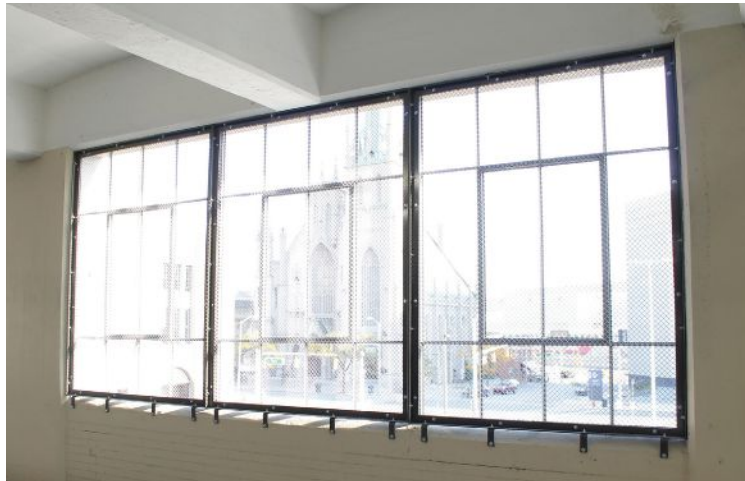
BlackBerry restored 30,000 square feet of hot-rolled steel windows at the Detroit News Parking Garage. Photos by BlackBerry
