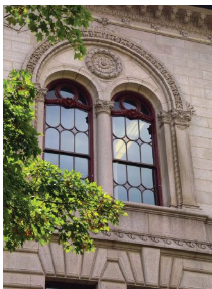
Kronenberger & Sons Restoration did restoration work at Worcester City Hall.
