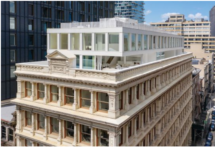
Clockwise from above, the two-story penthouse addition, cast-iron facade along Broadway, and indoor-outdoor living spaces enabled by full height sliding doors on the 8th floor.
