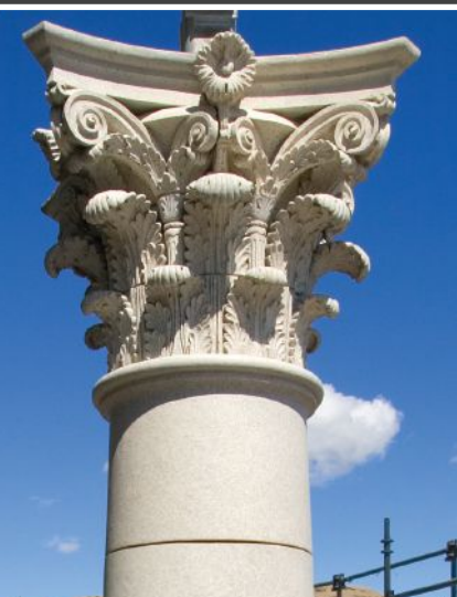
Utah State Capitol Dome Restoration
