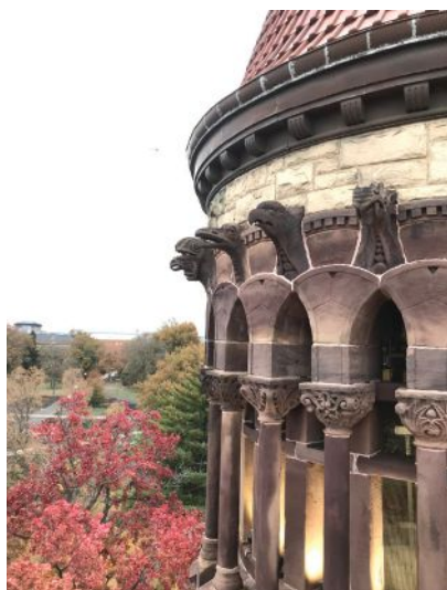
Orton Hall Columbus, OH EverGreene completed an exterior stone masonry survey in Oct 2018.
