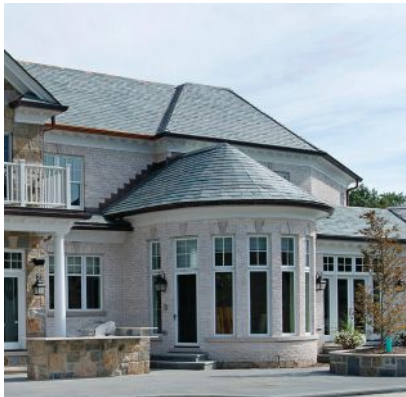
Greenstone's Non-weathering Gray / Green was the perfect choice to complement this elegant New England Colonial's stone exterior.
