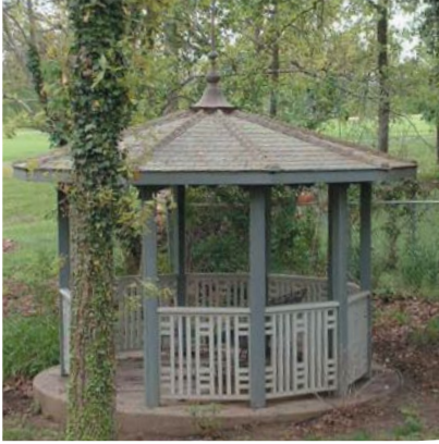
This gazebo features W.F. Norman's Style "A" shingles with its continuous hip finish and a custom-made finial on top.
