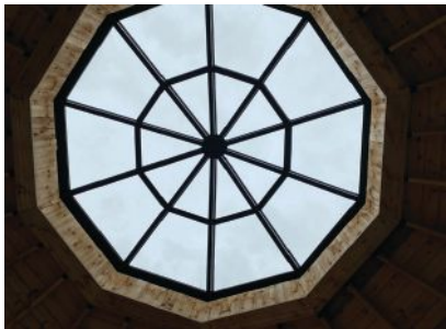
Glass House constructed this circular skylight.
