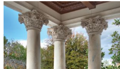
KEPCO+ restored the columns for the Utah's governor mansion.
