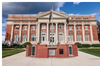
DeSoto County Courthouse, Arcadia, Florida, Historic Masonry Restoration was done by Graciano .
