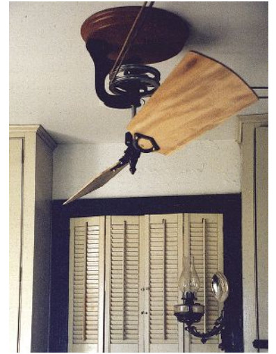
This belt-driven ceiling fan with solid-mahogany blades was supplied by Woolen Mill .
