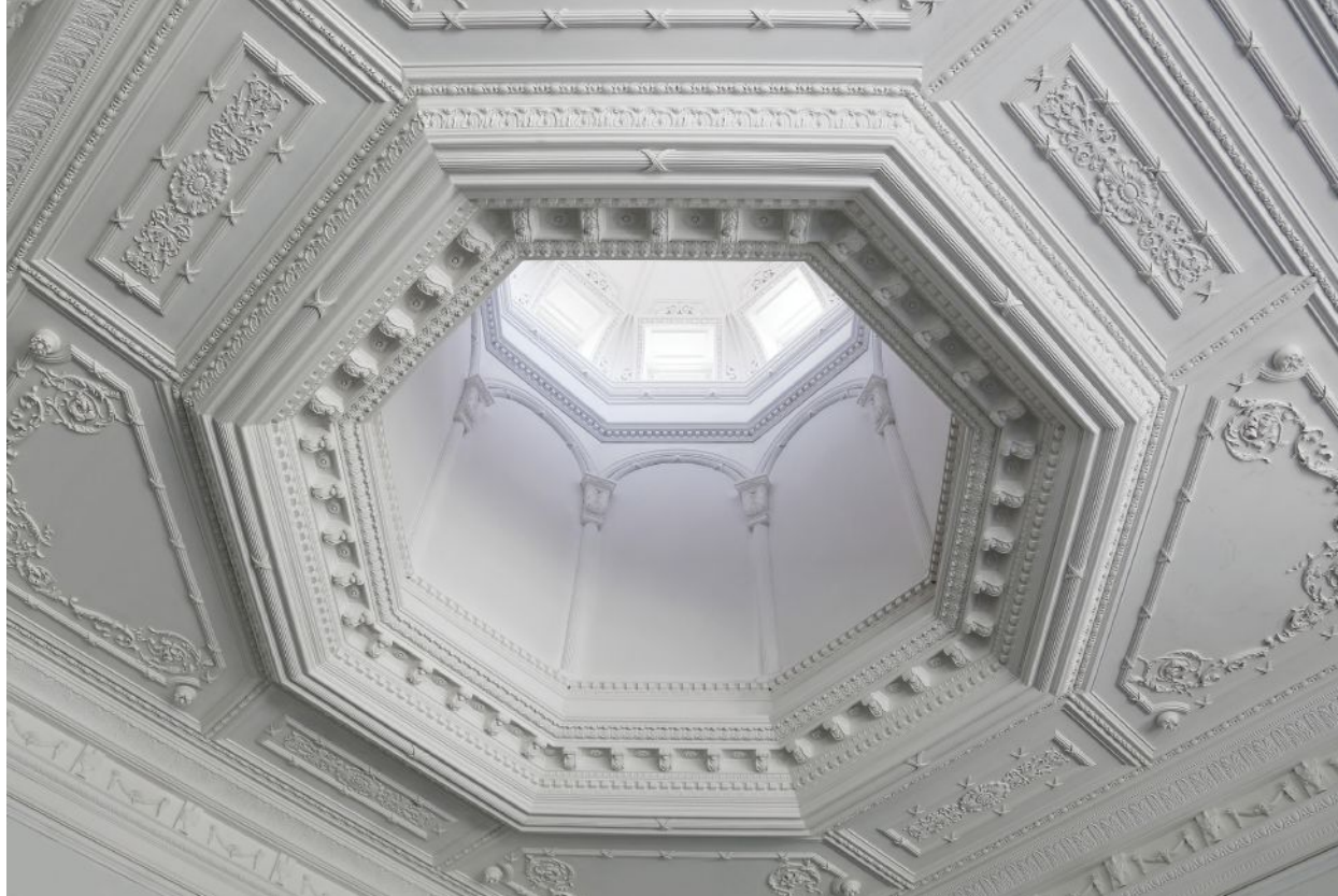
A skylight coffer is trimmed in plaster crown moulding from JP Weaver Company; the ceiling trims are from the company's Petitsin Line. Photo by Stephanie Croce
