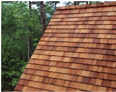
Western red cedar shingles from Ecoshel were used to create this roof.
