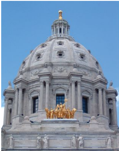
EverGreene took on regilding the exterior dome of the Minnesota Capitol building, which included rigging, stripping, and surface preparation as part of a larger effort to restore the capitol to its 1905 appearance.
