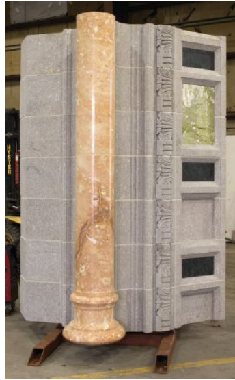
KEPCO+ attached three types of marble and Englishman Bay gray granite to a galvanized steel frame to create this detail.
