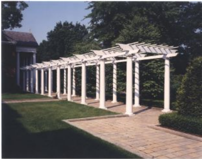
This pergola from Chadsworth was fabricated from cellular-PVC beams and rafters and PolyStone support columns.
