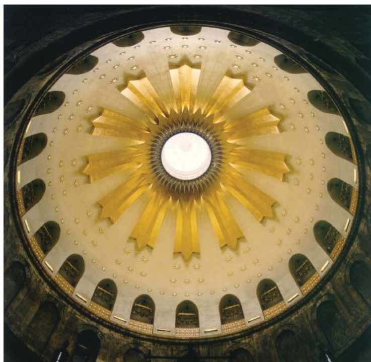
Above, at The Church of the Holy Sepulchre in Jerusalem, The Gilders’ Studio applied a linear textured pattern to the main rays, which were gilded with 23-karat gold leaf as were the stars and rings above it. The team also restored the circa 1869 gilding on the balustrades with 23-karat and 12-karat gold leaf.
