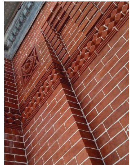
Left, Long Island's Montauk Lighthouse was repointed with Lancaster Lime Works' carbonating lime putty mortar.
