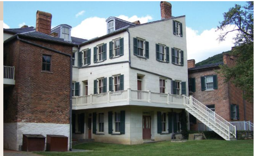
The restored Doran Block of historic buildings in the park.
