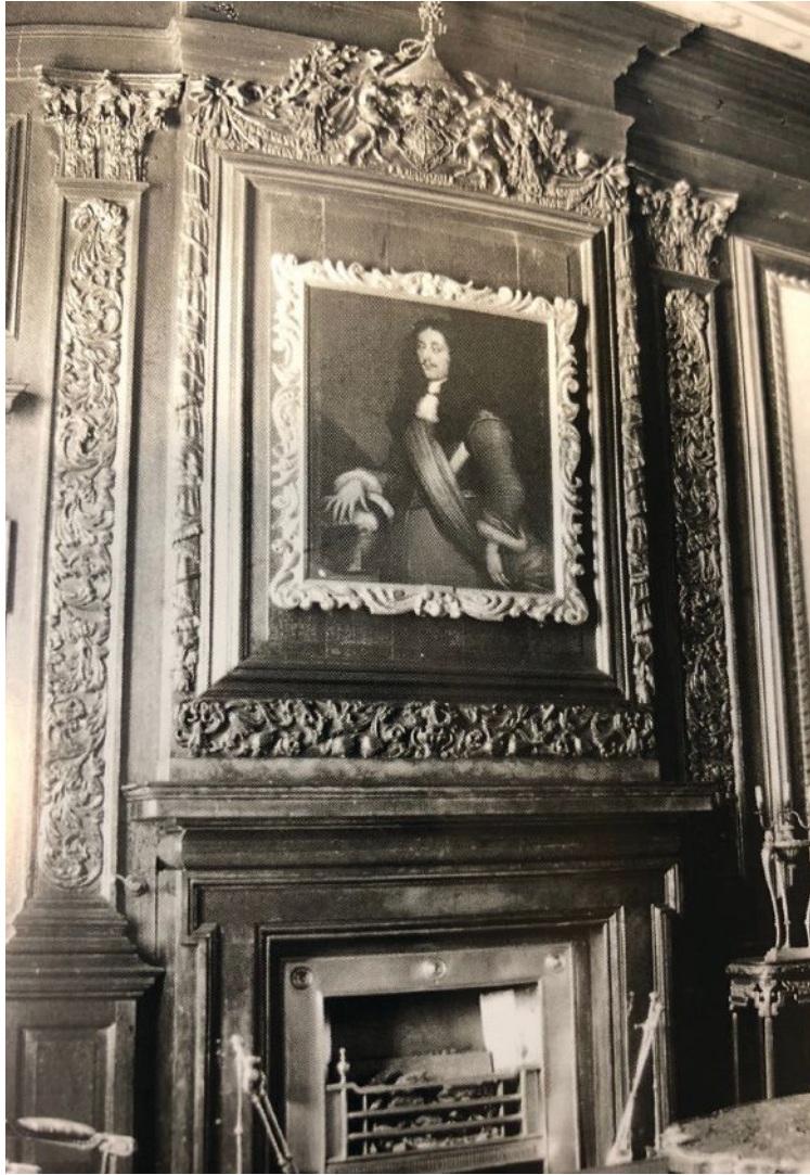
Clockwise from above, the original fireplace in Hamilton Palace, Scotland. The mantel frieze had been destroyed, and the mantel had been broken into several parts. The mantel leg before and after. The newly installed mantel with part of the remade frieze.
