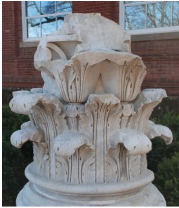
LEFT TO RIGHT: An original capital survivor from the 1895 fire; clay model of the upper portion on a reconstructed marble quarter capital; the final capital.
