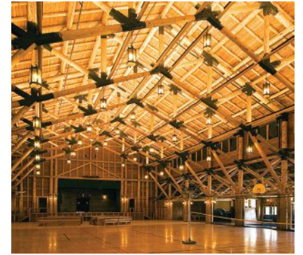
The restoration and replication of 216 Gothic-style pendant lighting fixtures from Yellowstone National Park's Old Faithful Lodge was performed by Grand Light .
