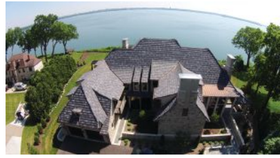
Lukis Restoration completed this project.
