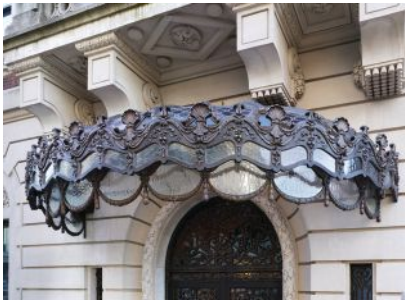
Kreilick Conservation worked on the Cooper-Hewitt Entry Canopy.
