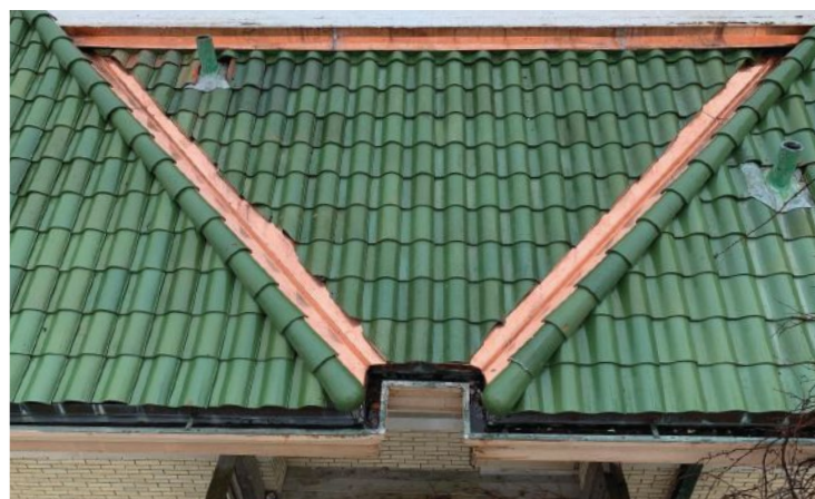
Lukis Restoration Co.: Left, Lukis Restoration supplied the new copper gutters, window flashings and flat roof for this house and re-laid sections of its concrete tile. Above, Lukis also re-laid sections of clay Spanish tile and added new copper flashings and a new flat roof above. Right, in addition to fabricating and installing new copper gutters, Lukis Restoration re-laid a section of the slate roof. Photos by Lukis Restoration Co.
