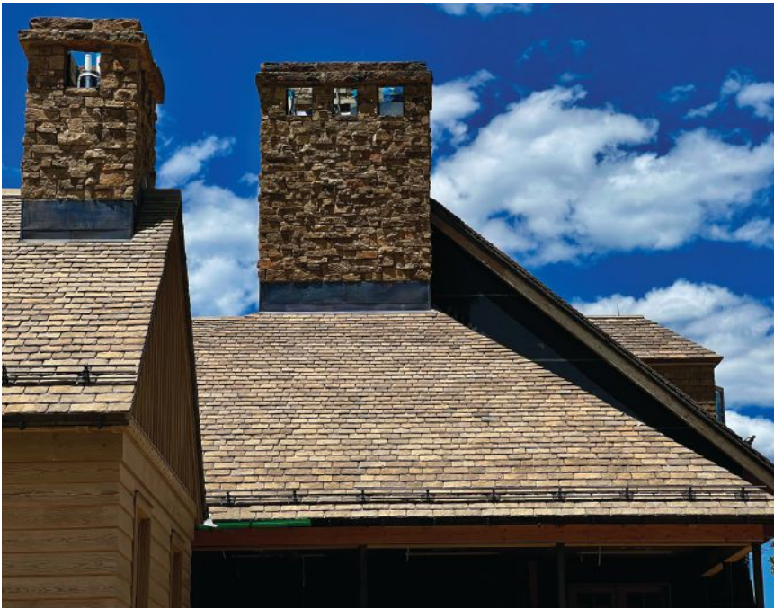
Northern Roof Tiles US: Above, manufactured in England and sold exclusively in North America by Northern Roof Tiles US, Cotswold Conservation is a cast stone replica that retains the natural stone's color and texture while combining modern installation methods. This installation is in Colorado. Right, English shingle tiles from Dreadnought Roof Tiles in England used for a project in Colorado. This roof is a blend of Staffs Blue Rustic and Dark Heather Rustic. Bands of ornamental tiles were included. Below, traditional pan and cover tiles in a wide range of colors and blends that are suitable for installation throughout the northern United States. Photos by Northern Roof Tiles US Inc.
