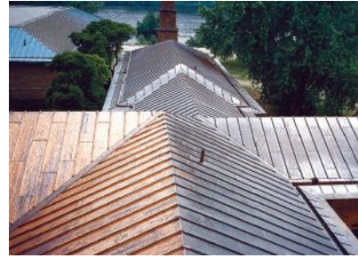
NIKO Contracting Co., Inc. installed this batten-seam and flat-lock copper roof.
