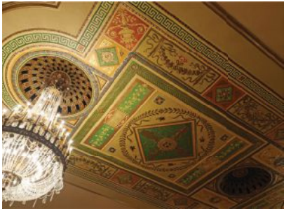
Conrad Schmitt Studios, Inc. was commissioned to restore damage to decorative finishes in the Crystal Ballroom of the Detroit Masonic Temple.
