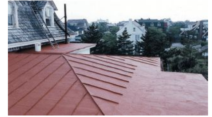
This metal roof has been treated with a waterproofing, elastomeric Acrymax coating from Preservation Products .
