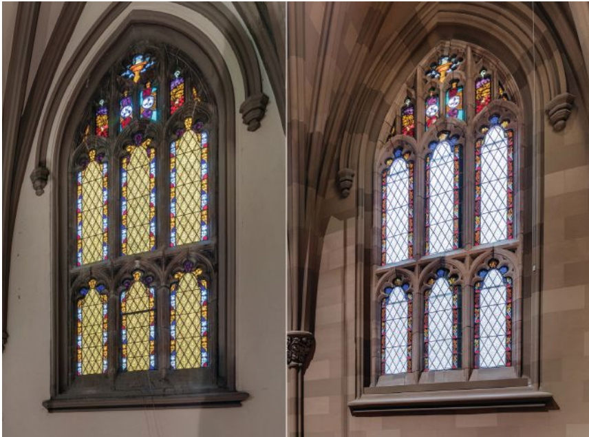
Above, clockwise: Non-historic yellow clerestory windows were replaced with historically accurate quarries that allow daylight to illuminate the restored faux-brownstone walls and ceiling. Photos by Colin Winterbottom
