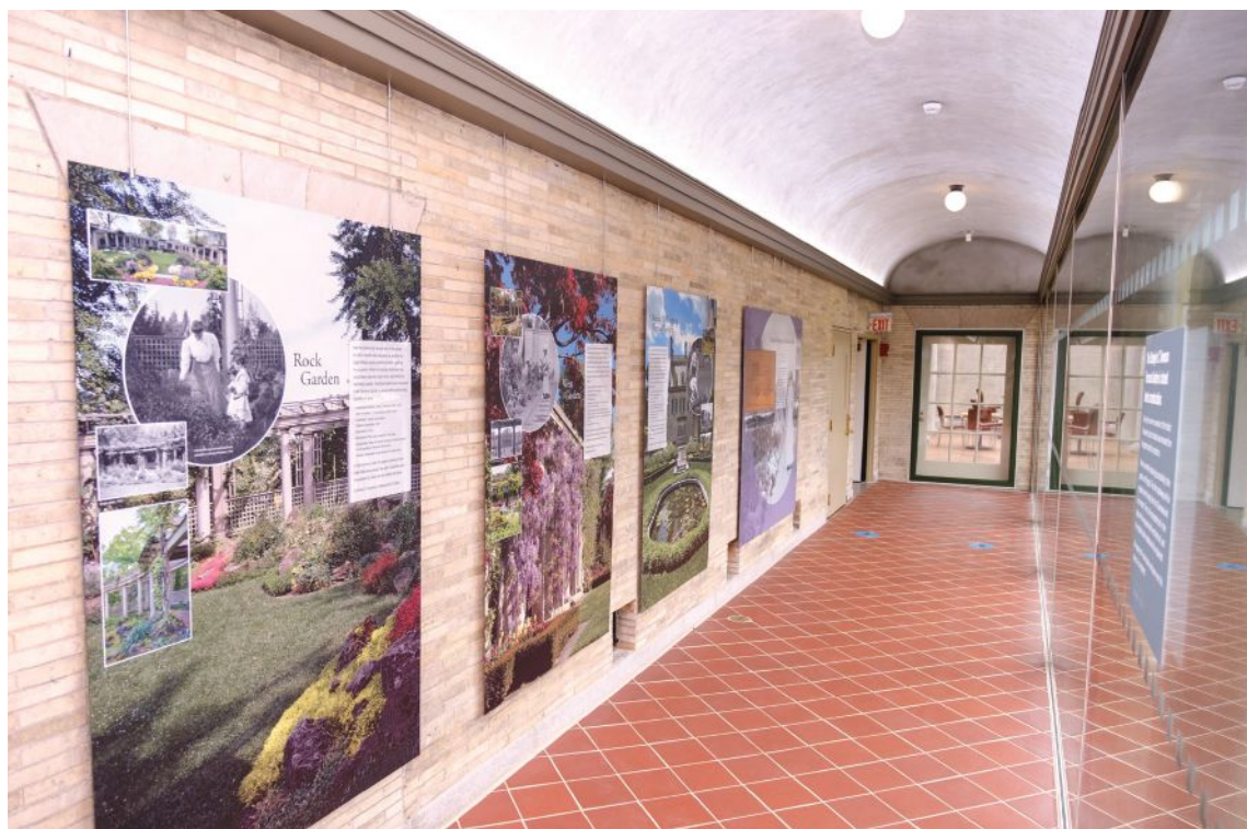
Above: Originally seasonal, the multilight panels became fixtures in the building’s architecture but performed poorly. Right: New insulated glass panels and a quarry tile floor bring year-round comfort to the colonnade.
