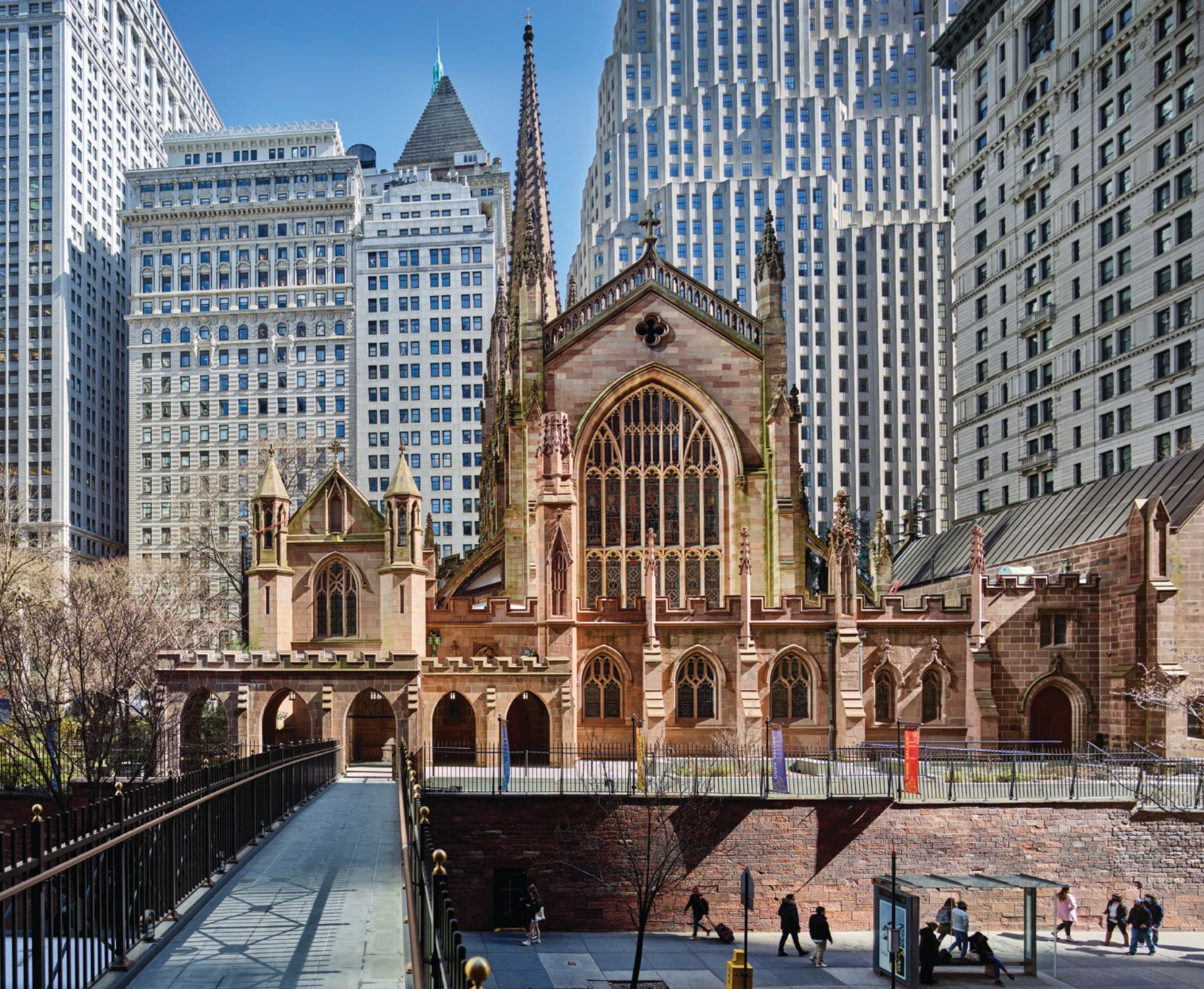
A new, accessible bluestone terrace wraps around the back of the church. A new brownstone loggia bay, matching the original, shelters a stair at the northwest entrance. Photo by Christopher Payne/Esto
