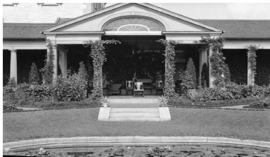
ABOVE: With a new insulated glazing system, the restored colonnade presents an open view of the garden and climate controlled passage to the Museum at right. LEFT: The colonnade in 1907—all limestone columns and all open.
