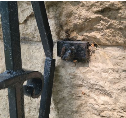
Above Left and clockwise: West Gate, Winnipeg, Manitoba. Three stone and wrought iron fences with light fixtures were built at the entrances into Armstrong’s Point, a 1911 gated community. Wrought iron light fixture atop the West Gate stone pedestal. A mild steel block was welded to the wrought iron member. Galvanic corrosion caused failure. Where the anchorage of the wrought iron has failed, do not repair with concrete. Its alkalinity will cause further corrosion, and the concrete will shrink, leaving small gaps where water will enter. Wrought iron corroding due to failure of the coating followed by environmental exposure of the iron.
