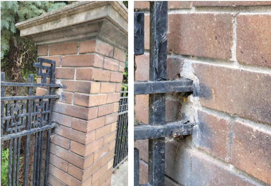
When the existing wrought iron has gaps or poor joints, they can be filled with red lead paint.
