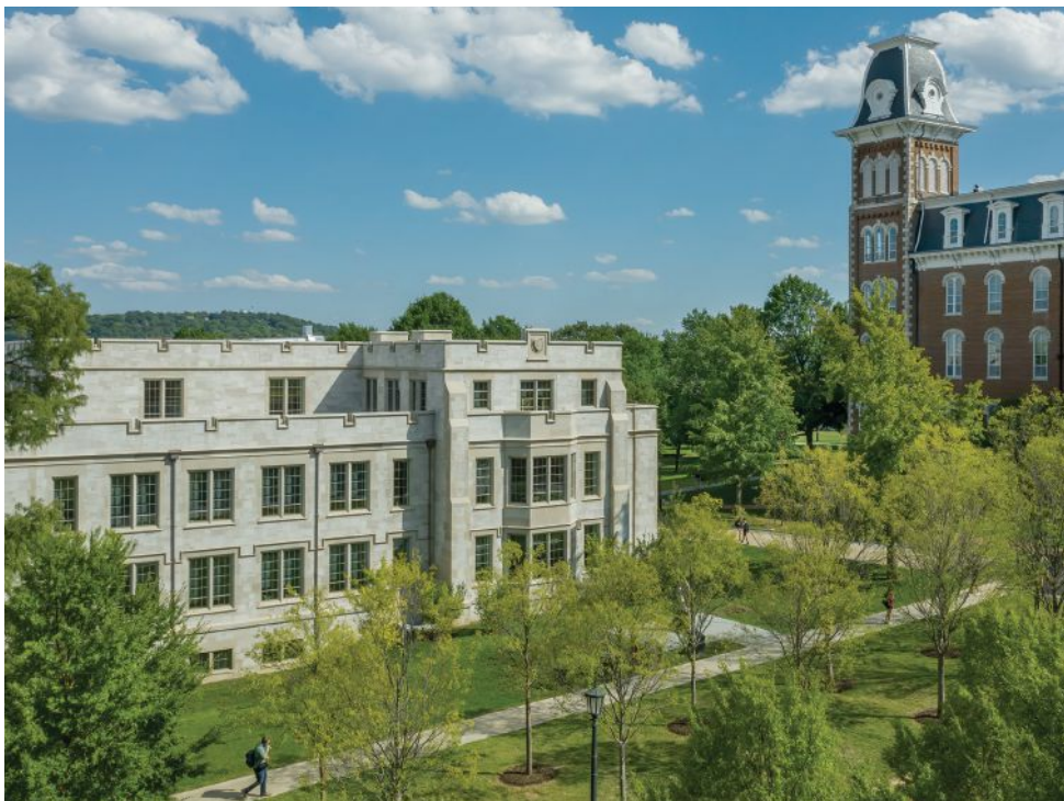
Above, west elevation. Right, the Batesville limestone on the center's facade is from the same quarry that supplied the quad's original buildings. The trim is Indiana limestone.
