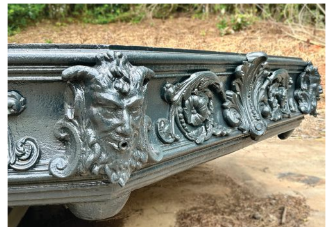
Robinson Iron disassembled the Court Square fountain for rehab in Alexander City. Fresh prime protects ornate cast iron in the shop. Above: Parts like basin got minor repairs before final finishes.
