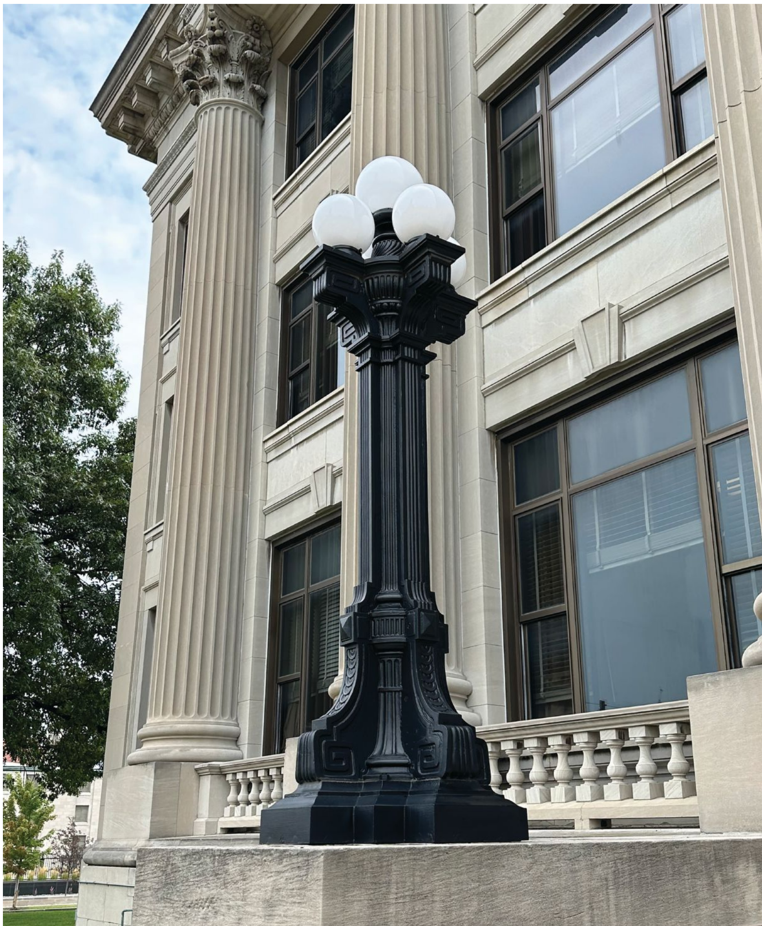
Illinois State Police Central Headquarters - Exterior Lighting Restoration
