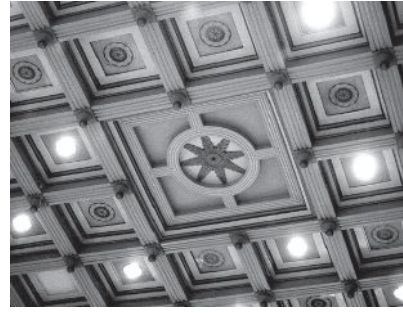
NIKO Contracting Co. 412-687-1517; Fax: 412-687-7969 www.nikocontracting.com Pittsburgh, PA 15213
