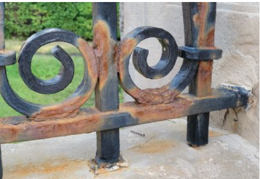
Above Left and clockwise: West Gate, Winnipeg, Manitoba. Three stone and wrought iron fences with light fixtures were built at the entrances into Armstrong’s Point, a 1911 gated community. Wrought iron light fixture atop the West Gate stone pedestal. A mild steel block was welded to the wrought iron member. Galvanic corrosion caused failure. Where the anchorage of the wrought iron has failed, do not repair with concrete. Its alkalinity will cause further corrosion, and the concrete will shrink, leaving small gaps where water will enter. Wrought iron corroding due to failure of the coating followed by environmental exposure of the iron.
