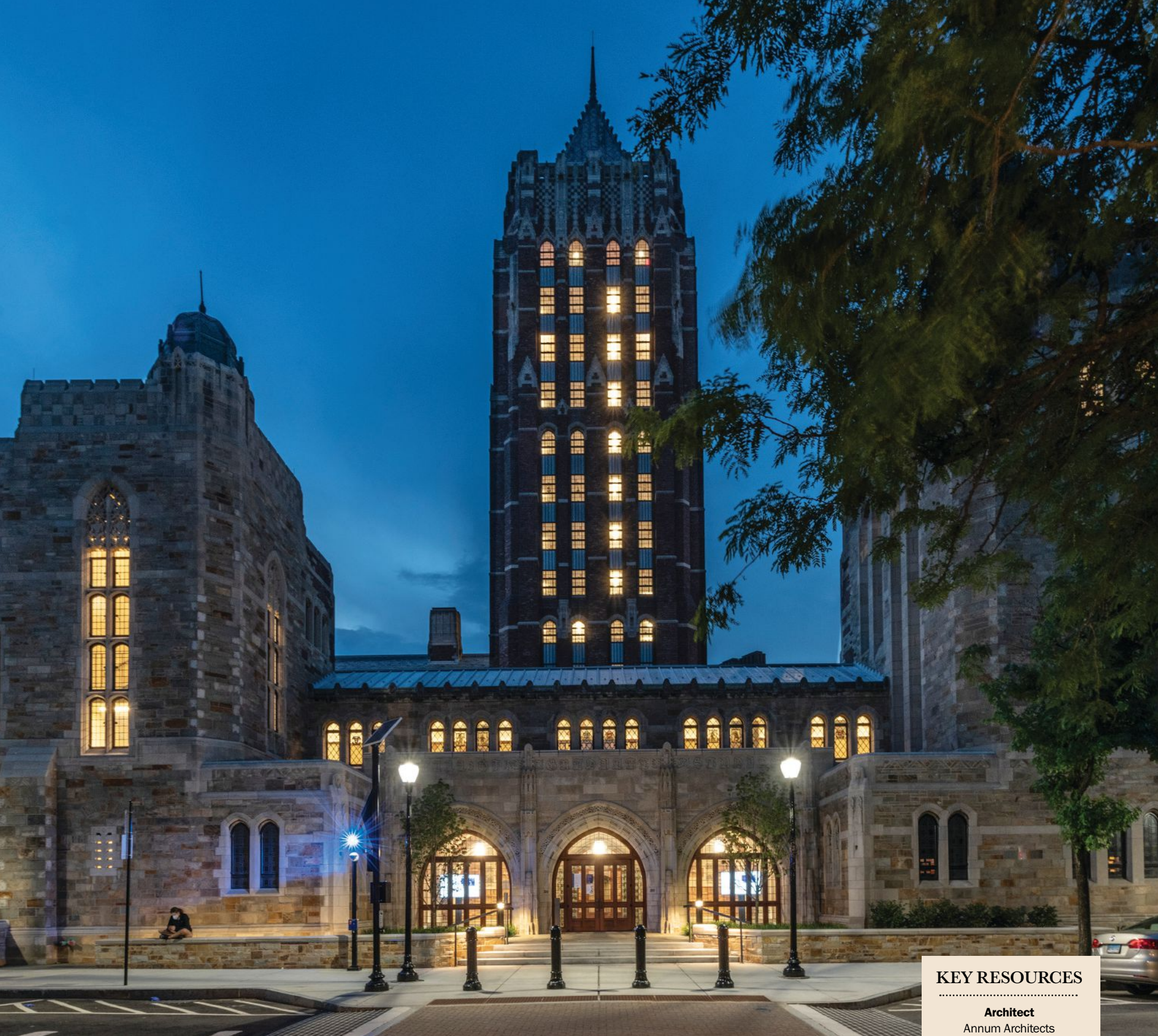
Among the broad palette of materials around the complex that were either cleaned or restored are stonework, such as the carved artisanal figures near the entrance on the first floor. The original front gates, cleaned and reinstalled, were produced by legendary blacksmith Samuel Yellin.
