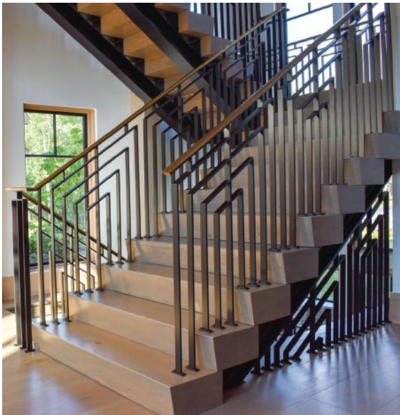
Compass Ironworks fabricated this transitional staircase composed of rustic Douglas fir treads (above) and contemporary railing design (right) with bronze cap.
