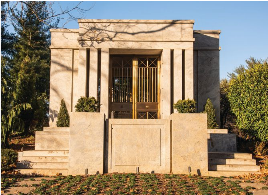
For the custom solid metal gates of a Private Monument, Wiemann used C38500 architectural bronze, an alloy popular for doors and handrails. Grilles are solid metal with a light patina. UV-stable lacquer coats the metalwork to resist weathering and maintain the smooth, satin aesthetic.
