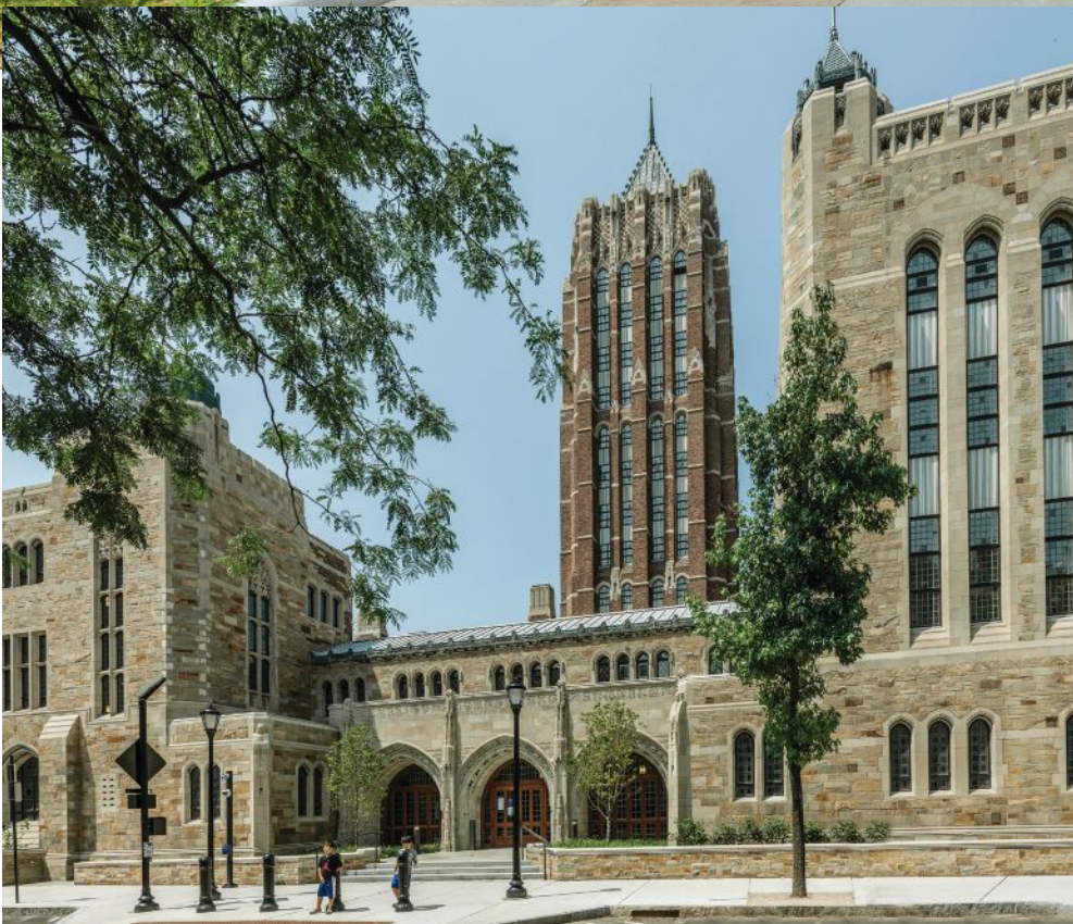
ABOVE: This central courtyard bounded by four sections of a Quadrangle – a pet Rogers plan – is, in effect, the roof of a 13,000 sq. ft. underground building holding the lecture and screening halls. LEFT: The 14-story Swensen tower, built with an early, unique curtain-wall system, was originally dorm rooms and completely rethought.
