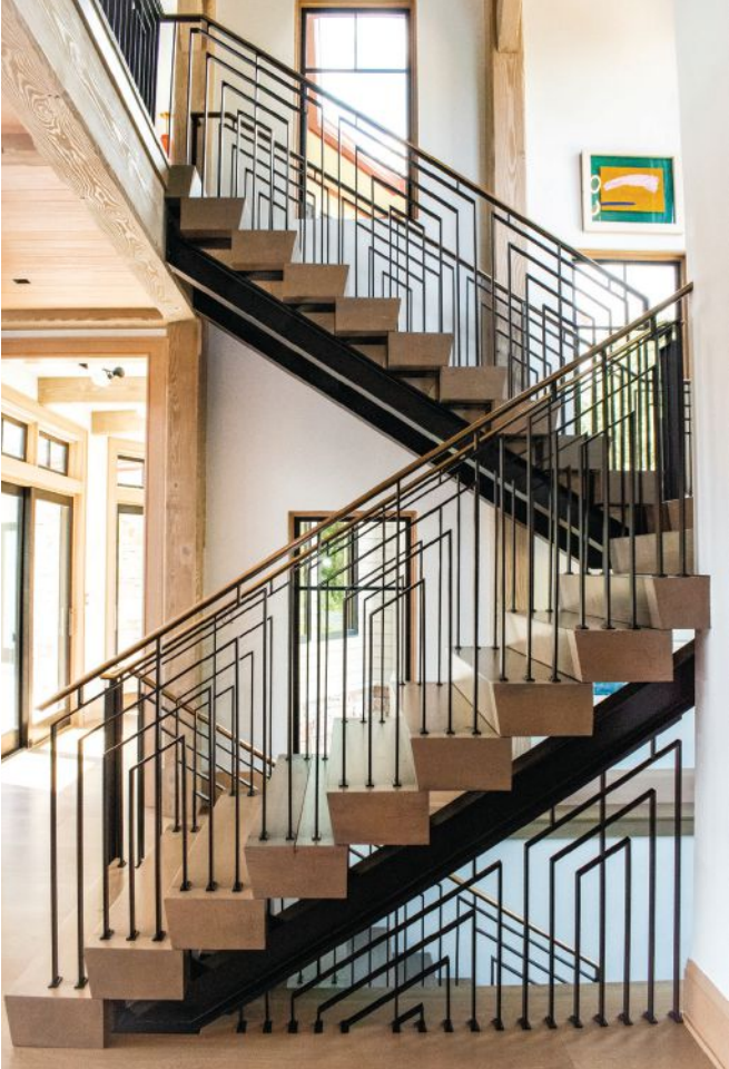
Compass Ironworks fabricated this transitional staircase composed of rustic Douglas fir treads (above) and contemporary railing design (right) with bronze cap.
