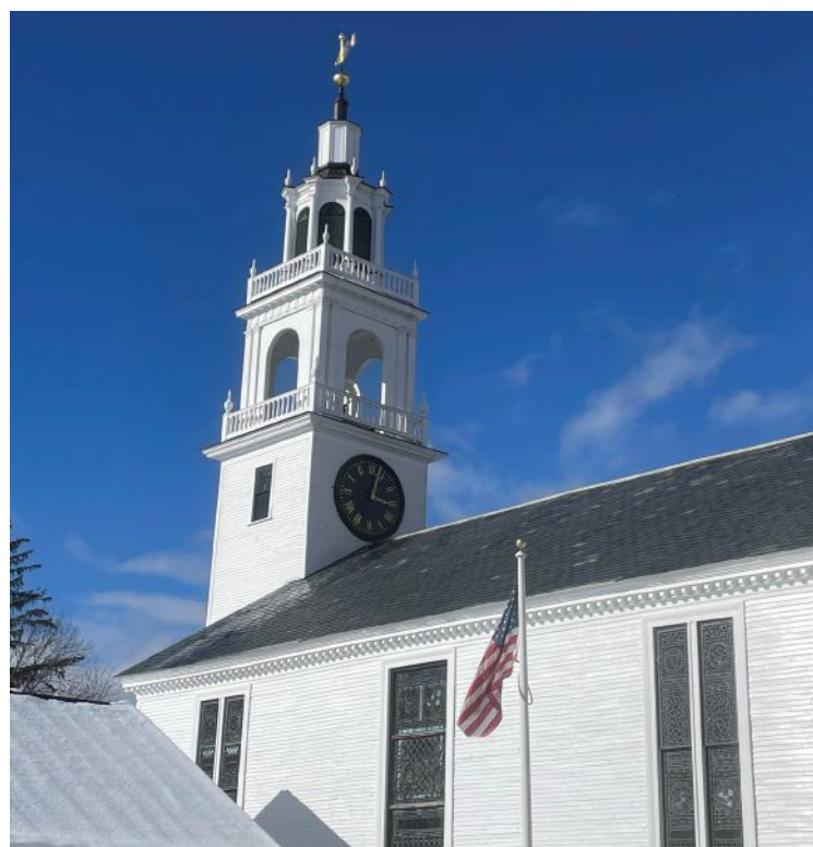
The First Parish Congregational Church in East Derry, New Hampshire, was one of Preservation Timber Framing's projects. Photo by Preservation Timber Framing
