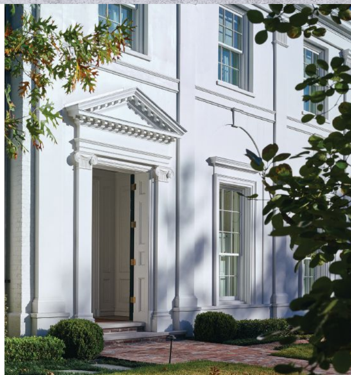
Entry portico at a new Regency-style house in River Oaks, Houston, Texas
