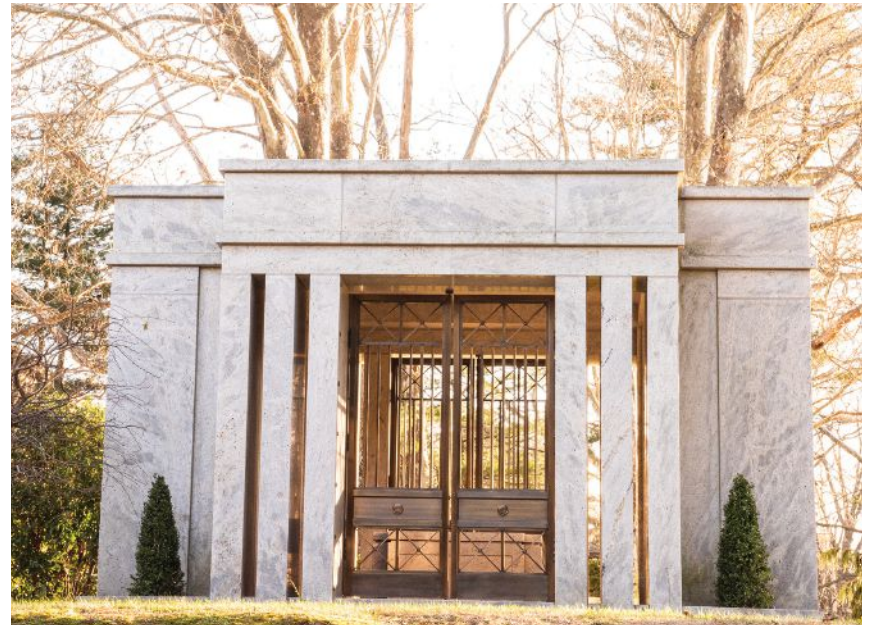
For the custom solid metal gates of a Private Monument, Wiemann used C38500 architectural bronze, an alloy popular for doors and handrails. Grilles are solid metal with a light patina. UV-stable lacquer coats the metalwork to resist weathering and maintain the smooth, satin aesthetic.
