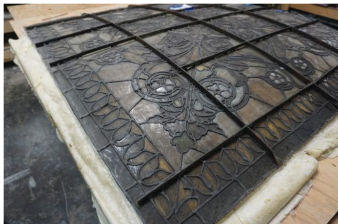
Right, one of the double-curved art-glass panels of the dome before restoration. Far right, recaming one of the art-glass pieces of the dome. Photos by Harboe Architects
