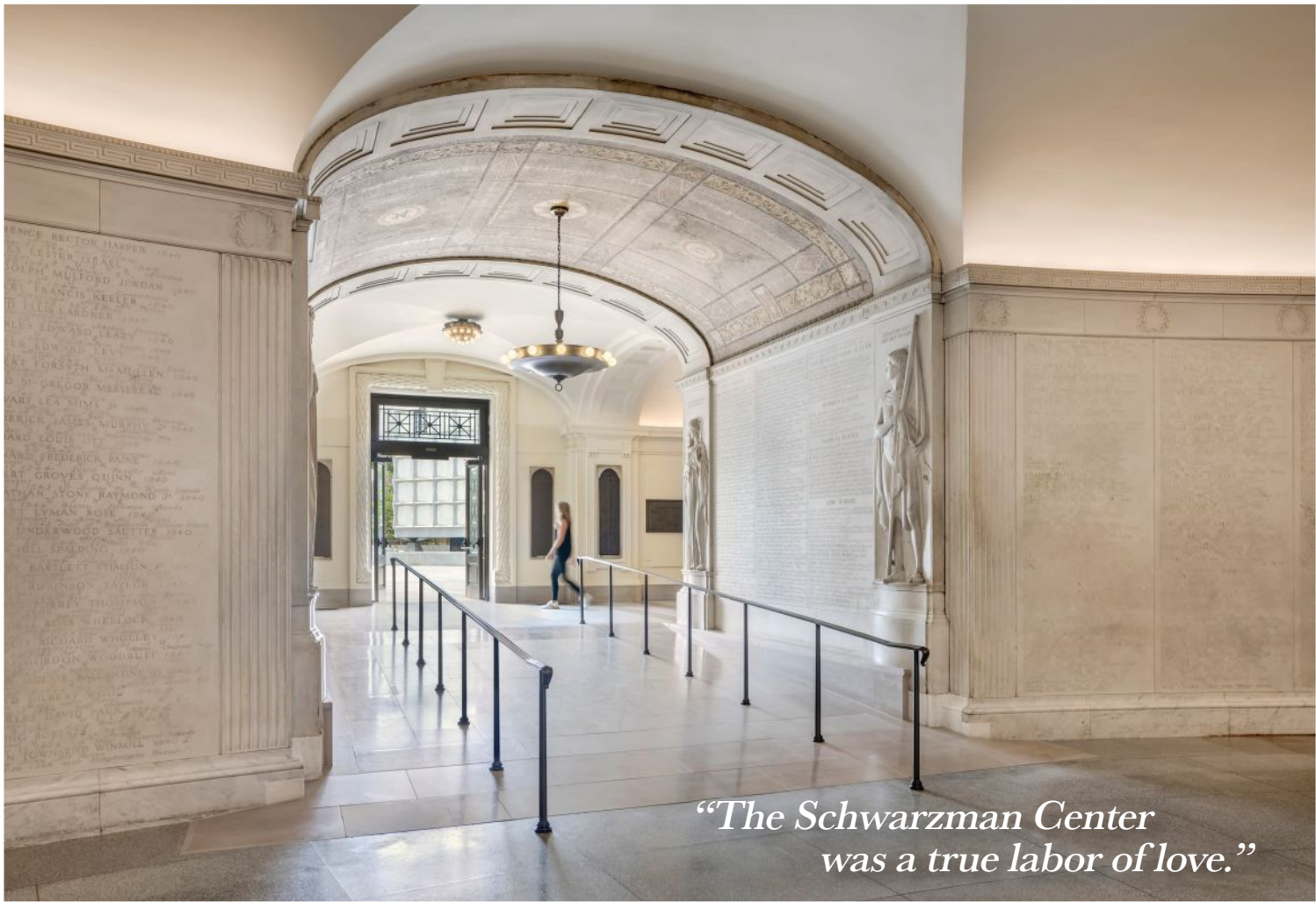
Left, the renovated rotunda gallery. The exterior of the rotunda restored to its original grandeur.
