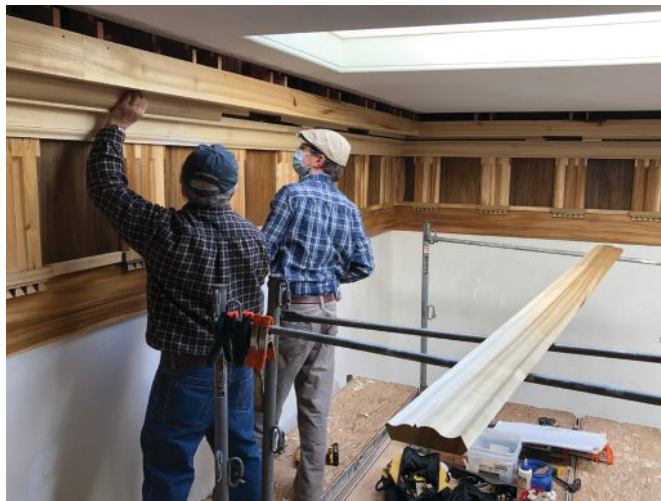
CLOCKWISE FROM TOP LEFT The craftsman paints a coat of varnish onto the entablature. Tuscan Order entablatures were installed in the entrance passage and in the bed chambers following Palladian proportions. All the interior trim was made by hand. The dining room's Doric Order entablature was made of four 20-foot segments.
