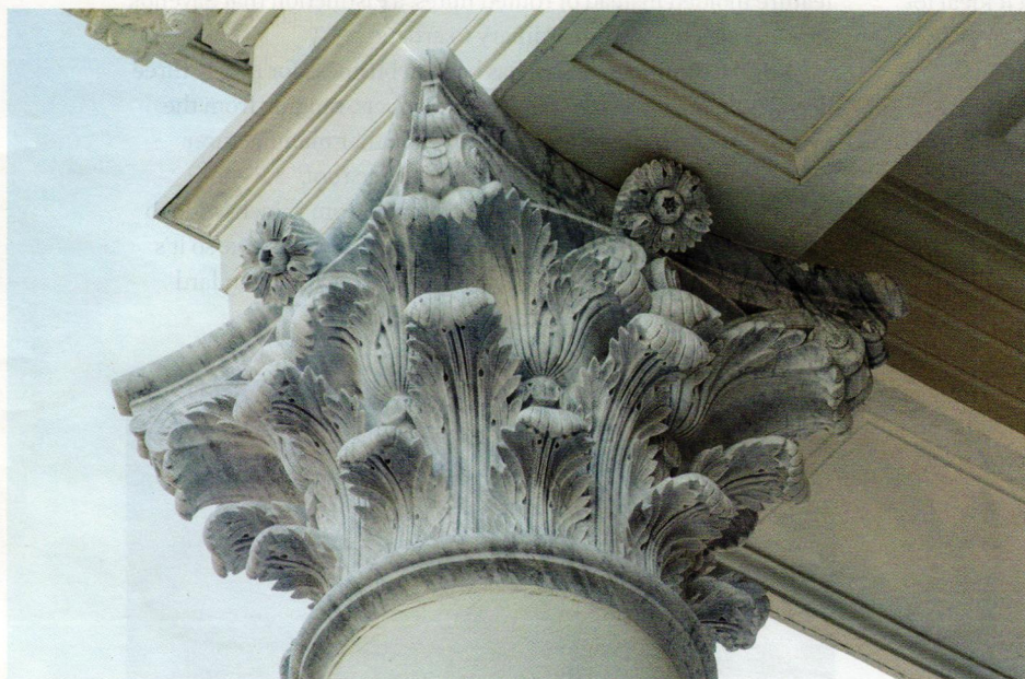
RUGO STONE, ABOVE Lacking any complete capitals, detailed photos, or original drawings, the Rugo team developed clay as well as plaster models based on remaining fragments of the old capitals, used 3D scanning, CNC machining, and hand carving to recreate the originals design.
