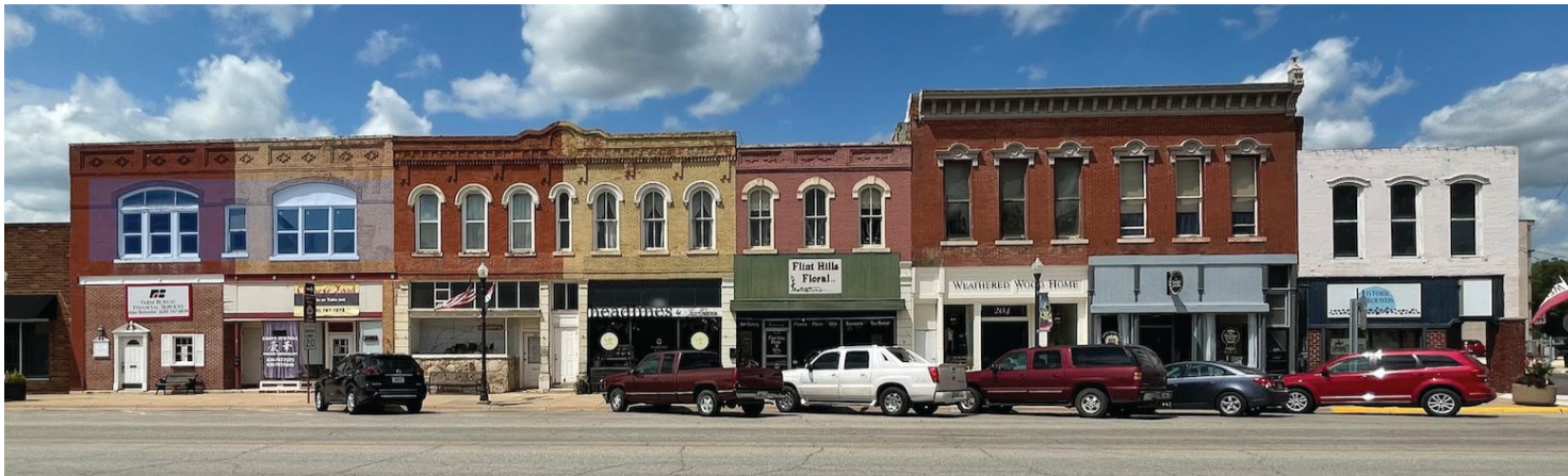
LEFT For main street buildings, narrow footplates, a lack of water for fire suppression, and egress limitations are among the conditions that can often be addressed by using one of the code compliance methods included in the model International Existing Building Code .
