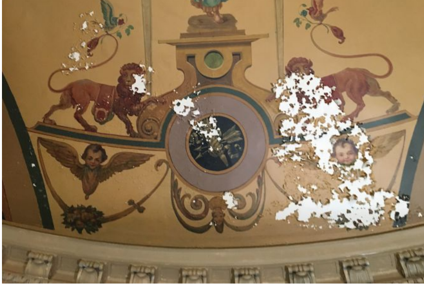
BELOW Scenes painted on canvas survived relatively unscathed except for being obscured by repeated shellackings. After painstaking shellac removal with swabs, the original colors of the 18th-century style murals sprang to life as if lit from behind.
