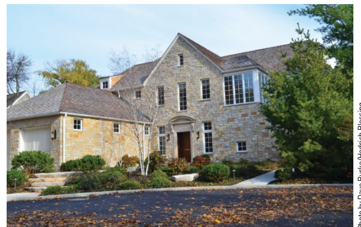
Photo by Dave Burke/Hedrich Blessing
