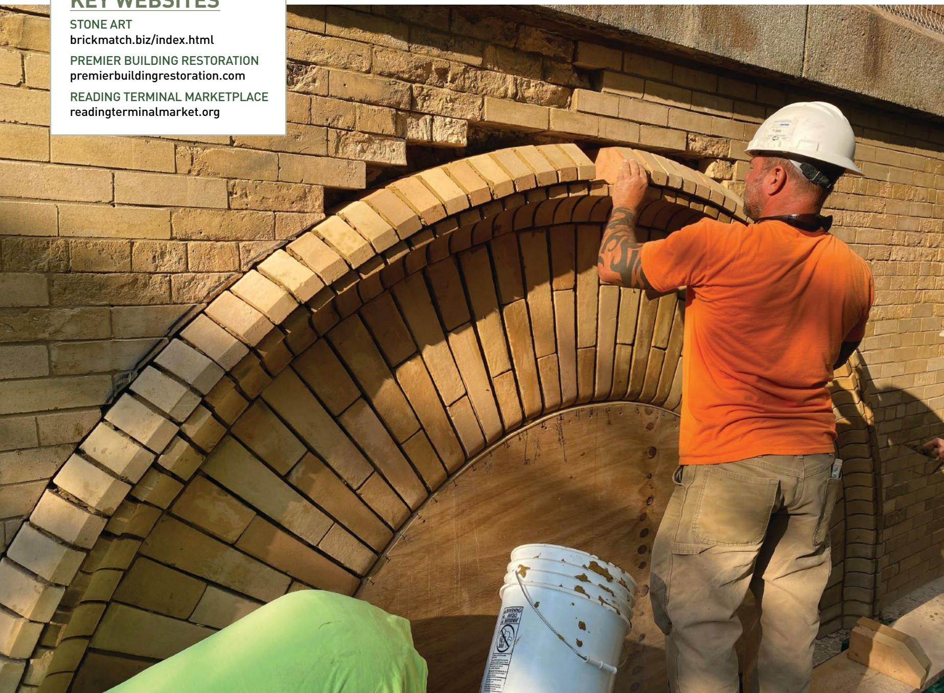
Photo by Premier Building Restoration
