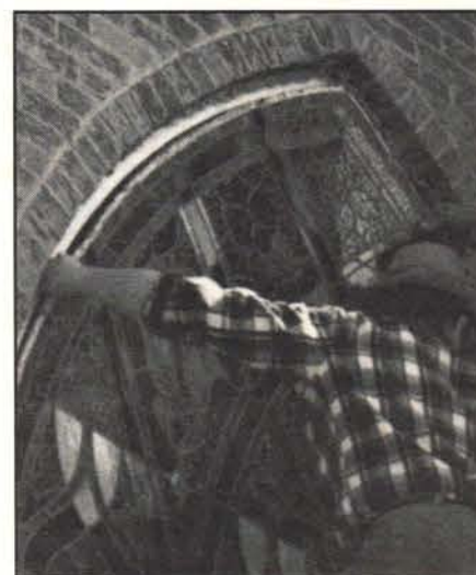
A crew from KAREN HENDRIX & ASSOC. removes a stained-glass panel that will be restored. Write in No. 271
