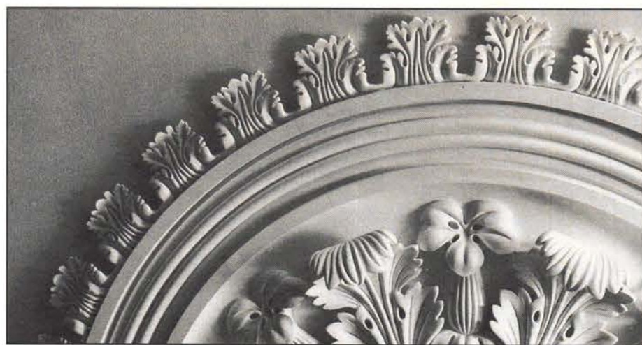
High-end casting jobs requiring meticulous attention to detail are the specialty of DAVID FLAHARTY, SCULPTOR. Flaharty designed and installed this period medallion on drywall using individually cast ornaments from Greek Revival originals.
