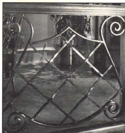
This custom-designed railing was forged, woven, and steel welded by ARCHITECTURAL INTERIORS BY SALAS & CO. The piece was doweled and epoxied into the wood railings and side walls. Write in No. 538
