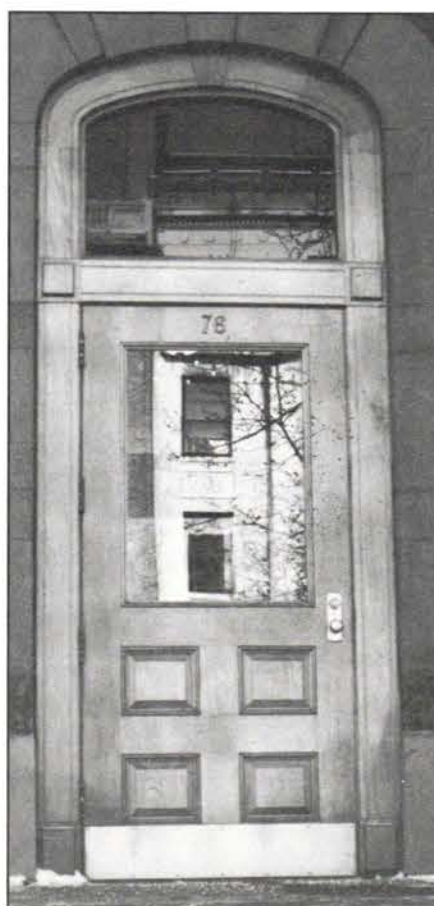
SOUTH SHORE MILLWORK made this sympathetic replacement door and transom for a Boston University entrance. The mahogany entry replaced an aluminum one. Write in No. 858
