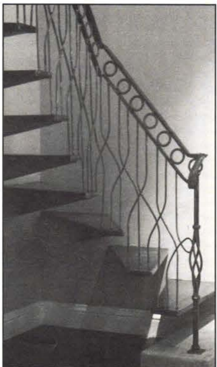
D.R. REIS METALWORKS fabricated this "designer's nightmare." A steel-with-pewter-finish bicycle spoke stair and rail was custom designed with stringers cantilevered from the wall and the top rail "floats" on the bent rods. Write in No. 363
