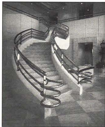
ZEPHYR METALS, INC. created this stainless steel Deco handrail system for a marble stairway for the Corporate Plaza Building, in San Jose.
