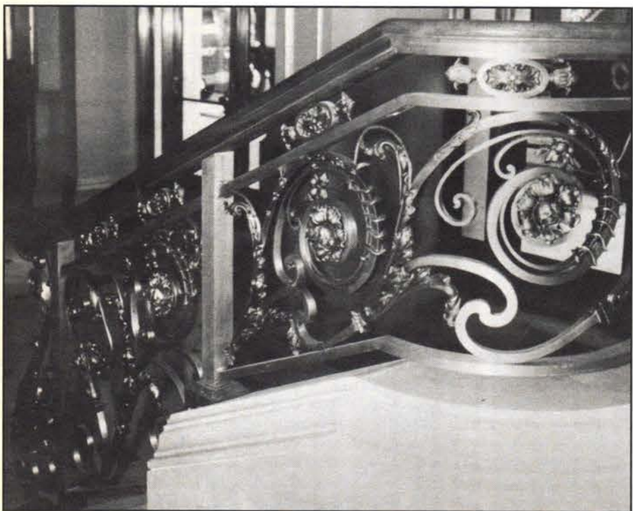
HISTORICAL ARTS & CASTING replicated all of the missing handrail at the c.1909 St. Regis Hotel, in New York City. The elegant body was cast in bronze and given a light antique green finish; the rail cap is mahogany. Write in No. 121
