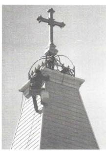
After reinstalling the cross that had been removed for gold leafing, a worker from JACK HASSLER CO. paints the cornice atop the steeple to complete the job. Write in No. 269
