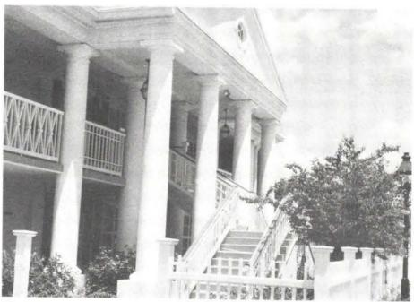
The joints on these GRC Doric columns are treated with a specially formulated exterior joint compound to achieve a monolithic surface. WEATHER ROK BY PLASTERGLAS, INC.
