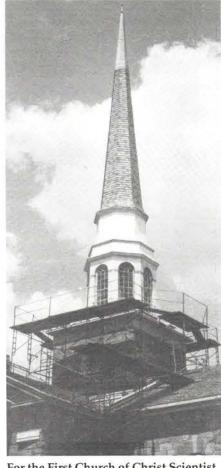
For the First Church of Christ Scientist, Montclair, N.J., ROGERS ROOFING fabricated and installed new copper cladding on the steeple, restored the steel windows, and painted the steeple inside and out. Write in No. 746
