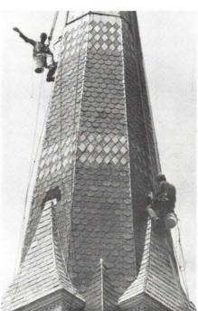
Fearless steeplejacks from YANKEE STEEPLEJACK CO. are replacing all the slate roofers and copper flashing on the spire of the United Church of Auburndale, Newton, Mass. Write in
