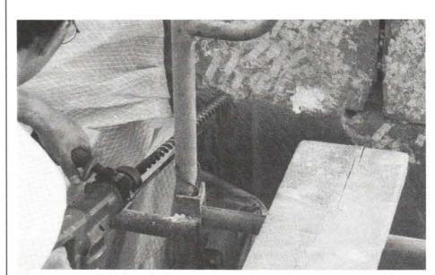
The innovative, British-made Cintec Harke stainless steel anchors are rather like large scale dentistry. A small hole is drilled into the damaged area and polyester-wrapped pins inserted — crossing each other like underpinnings. The polyester "sock" is then pumped full of grout, filling the sock from back to front.
