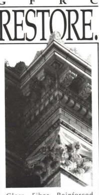
Glass Fiber Reinforced Concrete (GFRC) is ideal for building rehabilitation or retrofit projects. Its light weight minimizes the load added to the existing structure.
