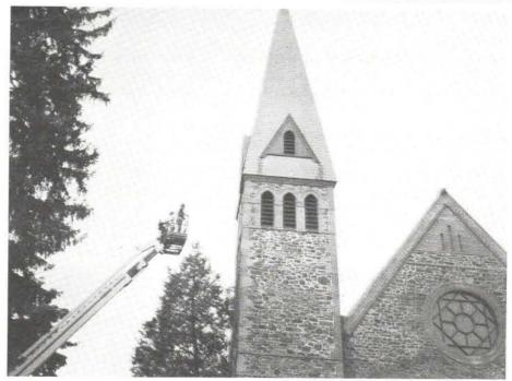
Instead of erecting scaffolding, CRL of Maryland used a cherry picker to inspect St. Stephen's Church and do 5,000 lineal feet of stone re-pointing and 3,800 lineal feet of brick pointing.
