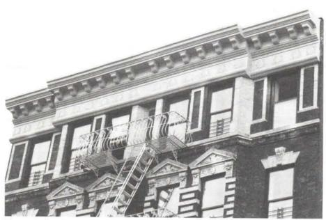
"Stuart Style" fiberglass cornice in New York City by ARCHITECTURAL FIBERGLASS CORP. Write in No. 640
