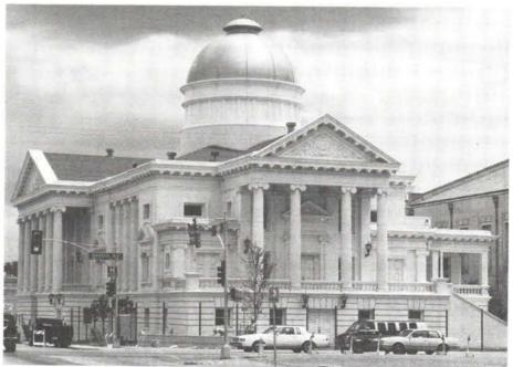
MOLDED FIBER GLASS fabricated this self-supporting FRP dome and columnenhanced base, which sits atop Criswell College. Write in No. 922
