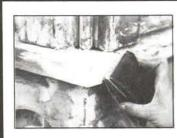
**LiquidWood** and **WoodEpox** give new life to severely rotted windowsills, sash, frames, shutters, columns, antiques, decorative wood elements. The Abatron system is especially valuable when original wood must be saved for historic reasons. LiquidWood consolidant reinfor-
