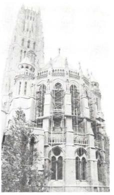
Extensive repairs to the magnificent stained glass windows in New York City's Riverside Church required, among many other things, the erection of 80-ft. scaffolding by ROHLF'S STAINED GLASS STUDIOS. Write in No. 624
