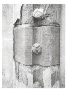
The center portion of the sandstone moldings surrounding a church entrance has been recreated in place using Jahn patching mortar from CATHEDRAL STONE PRODUCTS. Write in No. 380
