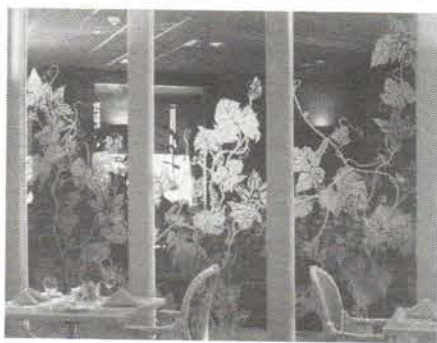
This grapeleaf motif has been acid etched on both sides of tempered glass panels and installed in a Winston-Salem, NC restaurant. NEWE DAISTERRE GLAS. Write in No. 313
