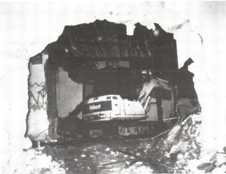
Demolition the hard way: The structurally unsound stage house had to be demolished by bringing equipment through a wall in the surrounding new construction.
