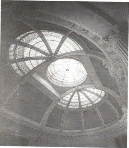
CUMMINGS STUDIOS replicated this ceiling in the rotunda of the Old Executive Office in Washington, D.C. using original drawings from the turn-of-the-century. The restored ceiling contains over 12,000 pieces of glass in a central conical dome flanked by 2 quarter-spheres. Write in No. 316
