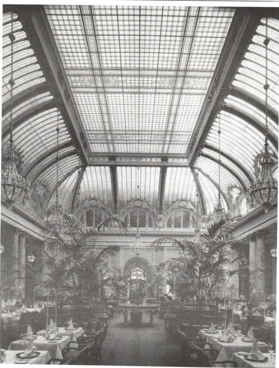
Restoration of the Garden Court ceiling in San Francisco's Sheraton Palace Hotel was done by REFLECTION STUDIOS. Over 8,000 sq. ft. and more than 30,000 pieces were either rebuilt or reproduced to the original 1909 design. They also designed and installed an earthquake protection system which individually suspends each panel. Write in No. 793
