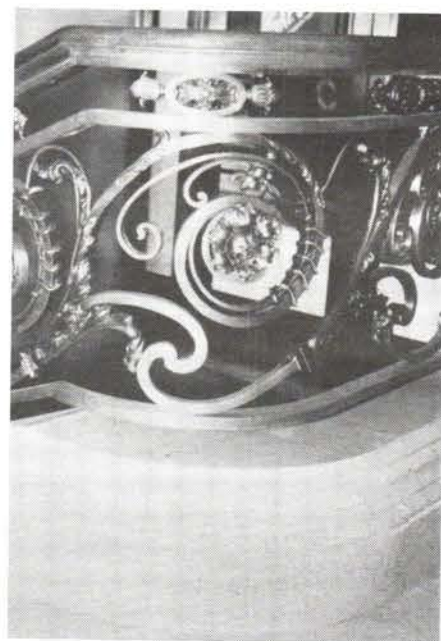
The bronze railings in the New York Sheraton St. Regis Hotel were cast by HISTORICAL ARTS AND CASTING using the lost wax process in order to capture the intricate detailing. Write in No. 121
