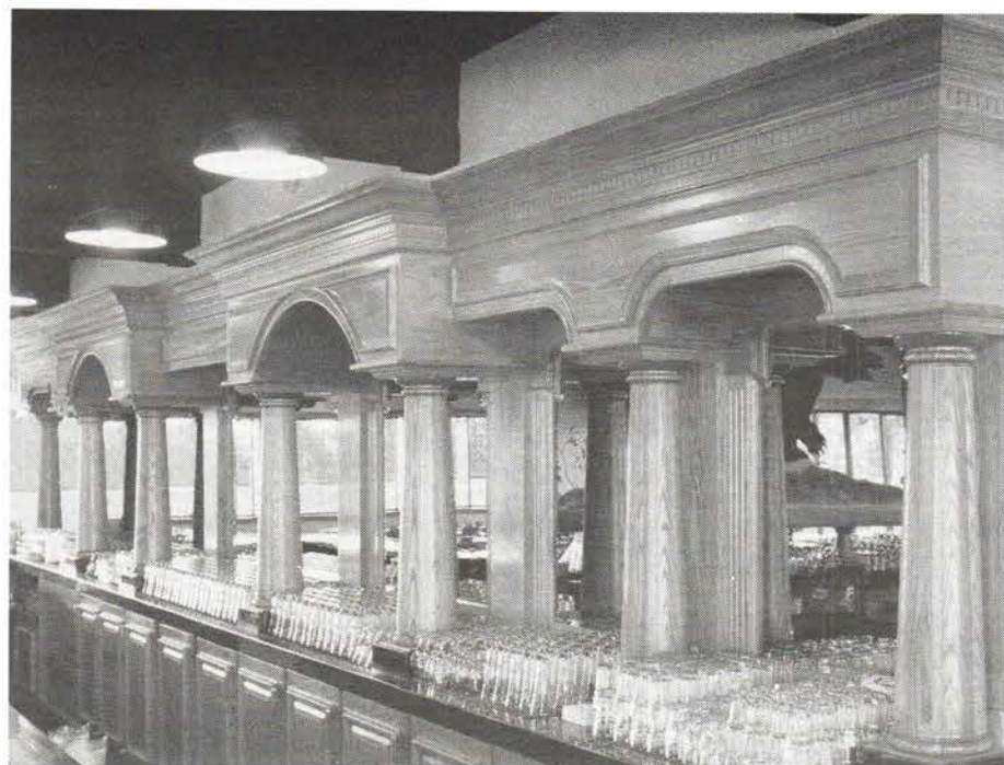
The superstructure and tapered columns of this back bar are made of red oak; the counter is black granite. POWELL CABINET & FIXTURE CO. Write in No. 852
