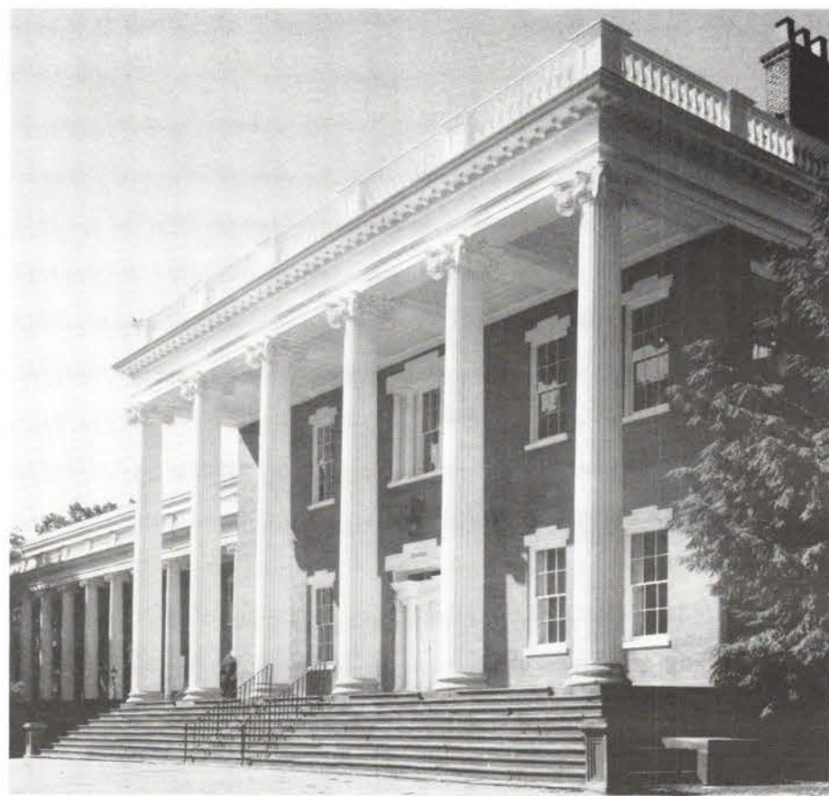
The facade of Drew University's Mead Hall, rebuilt with James G. Whildin, Jr., AIA of Spillman Farmer Architects: Much of its detail, including Corinthian columns and sidelit entry, miraculously survived a fire that started next to the front door and roared up the chimney-like space between the brick walls and the interior plaster. Photo: Jack E. Boucher
