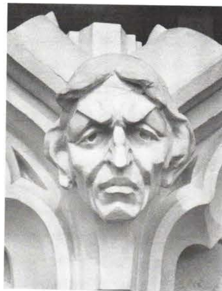
"Gargoyle Head" is one of 12,000 Gothic-style terra cotta castings replaced by thin-shell DESIGN CAST units, for a restoration in New York City.
