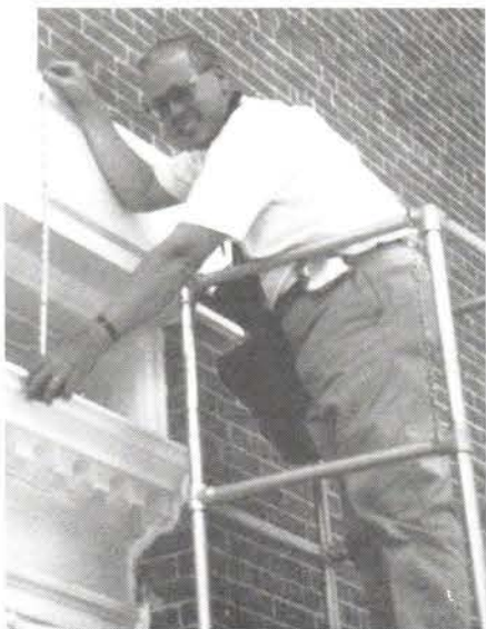
Jim measuring a doorway at Drew University’s Mead Hall for HABS-quality drawings of the structure. (It endured fire damage a few years later and was rebuilt based on Massey Maxwell’s drawings.) Photo: Anne Vytlačil, AIA
