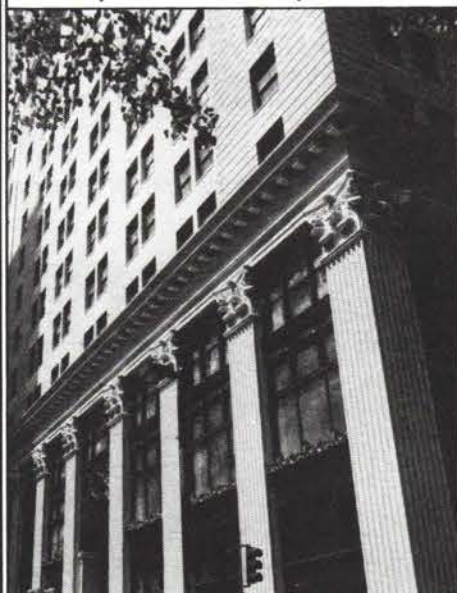
Restored facade of Widener Building. Capitals and horizontal ornamentation were made of fiberglass reinforced polyester resin in Polytek Rubber Molds.
