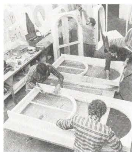
A glance into MIDWEST ARCHITECTURAL PRODUCTS' shop reveals craftsmen in the midst of fabricating reproduction windows for an historic renovation project. Write in No. 146
