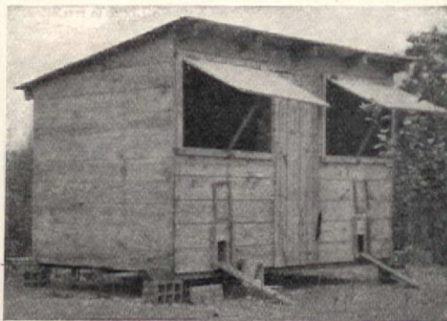
A Well-ventilated Colony House
