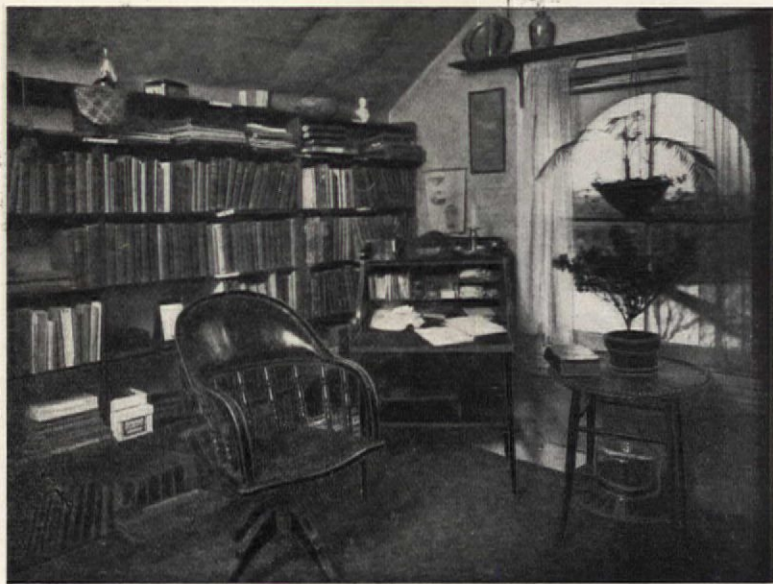
Two Cozy Attic Dens in Which Builders' Paper was Used Effectively to Make Ceilings and Walls. It was Tacked on the Exposed Beams
