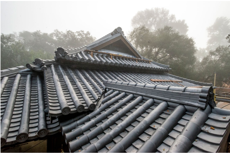
The roof tiles of the Japanese Heritage Shōya House.
