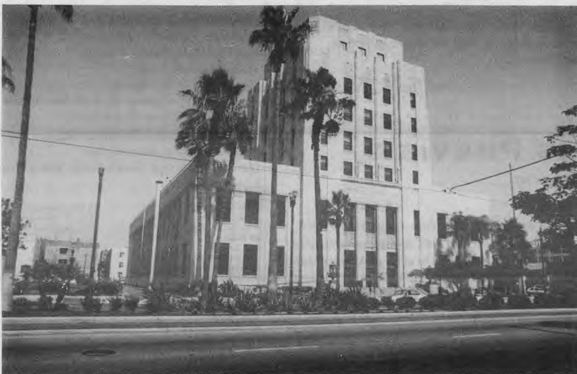
The 1931-32 Federal Building by Gordon Kaufman is now the Long Beach Post Office. (Photo: John Berley)
