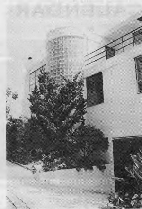
The Ulm House from 1937 exemplifies the Streamline Moderne style Merry Ovnick will discuss on July 9th.
