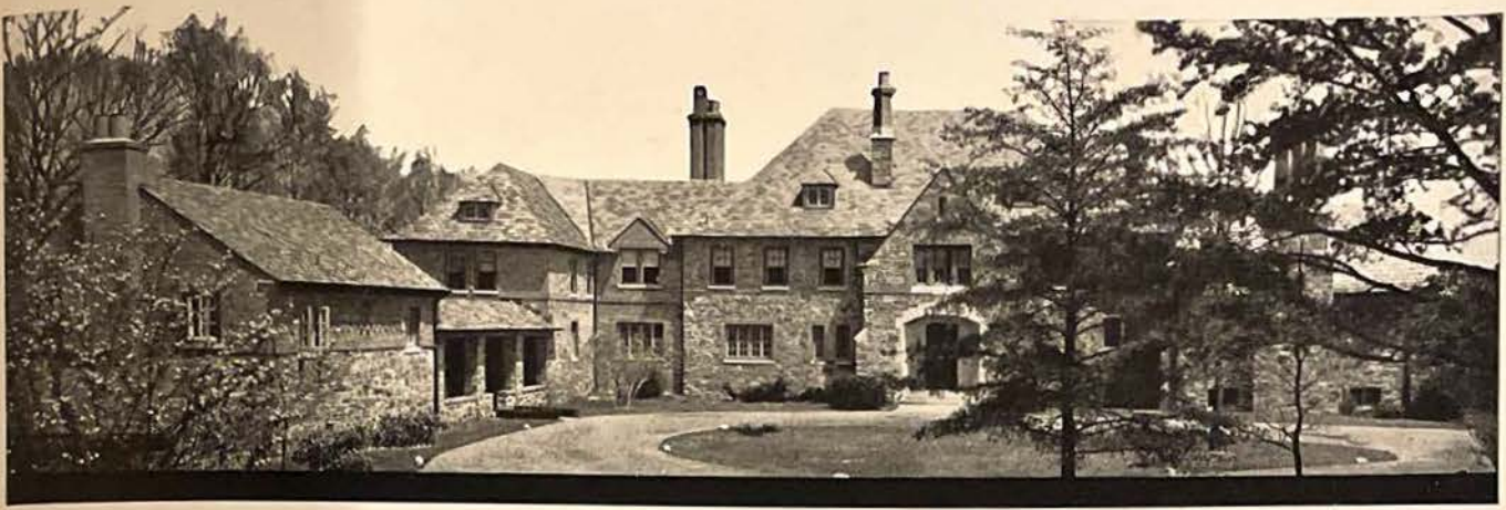
A 750-A intercommunicating system and eleven telephone outlets provide complete telephone convenience in the residence of Mr. Merle Thorpe, Rockville Pike, Montgomery County, Maryland. APPLETON P. CLARK, JR., Architect, Washington, D. C.
