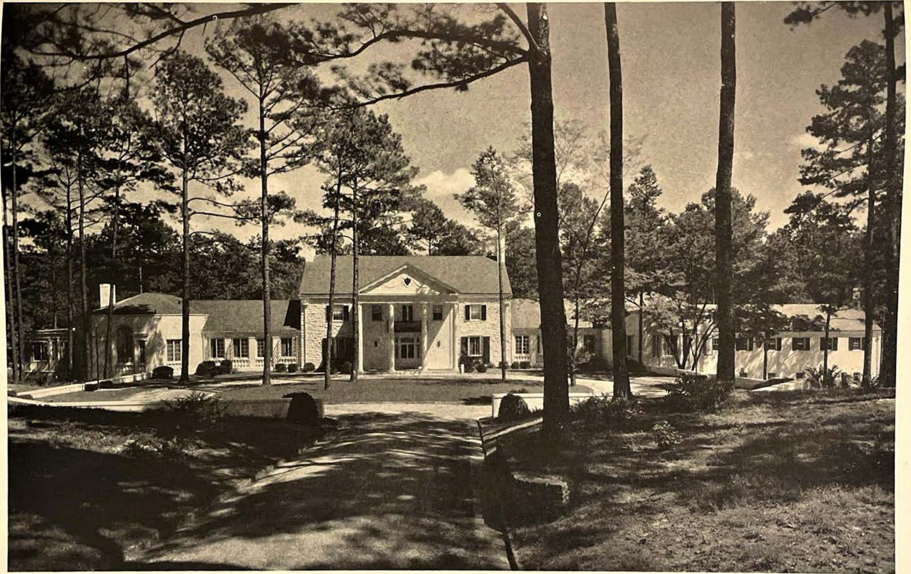
ENTRANCE FACADE, MOUNTAIN BROOK COUNTRY CLUB, BIRMINGHAM, ALA. AYMAR EMBURY, II, AND MILLER & MARTIN, ASSOCIATED ARCHITECTS
