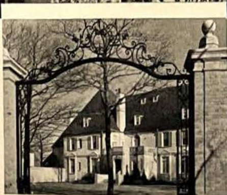
Residence of A. E. Cross, Evanston, Ill. Richard Powers, Architect
