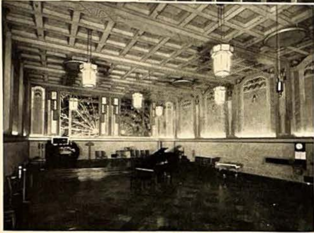
One of the broadcasting studios. Walls of two 6" layers of cinder concrete blocks separated by 2-inch air space
