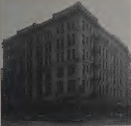
Milby Hotel, Houston, Texas Louis Glover, Architect Barber Plumbing Co., Plumbers Crane Co. and Standard Sanitary Mfg. Co., Jobbers
