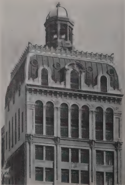
Illustrating 12th to 17th stories, incl., of the Security Building, showing the Terra Cotta trim
