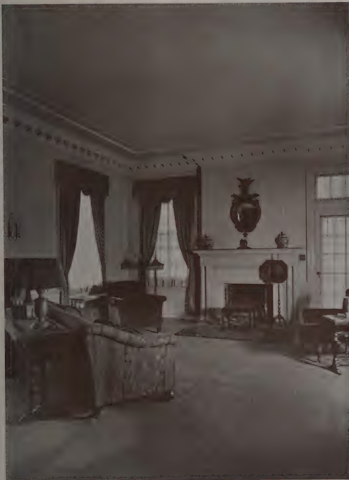
LIVING ROOM DETAIL HOUSE OF S. J. PATILLO, ESQ., ATLANTA, GA. PRINGLE & SMITH, ARCHITECTS
