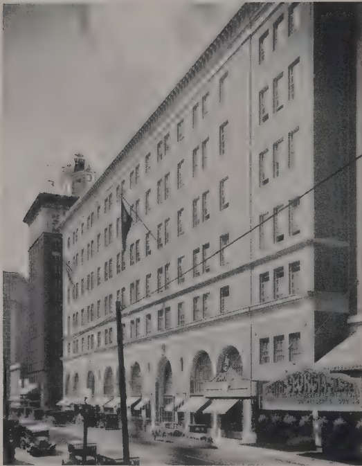
Macy's Department Store, Davison-Paxon Company, Atlanta, Ga. Equipped with Signal Call and Signal Fire Alarm Systems. Starrett & Van Vleet, Architects; Hentz, Adler & Shutze, Associate Architects; Harry Alexander, Inc., Electrical Contractors.
