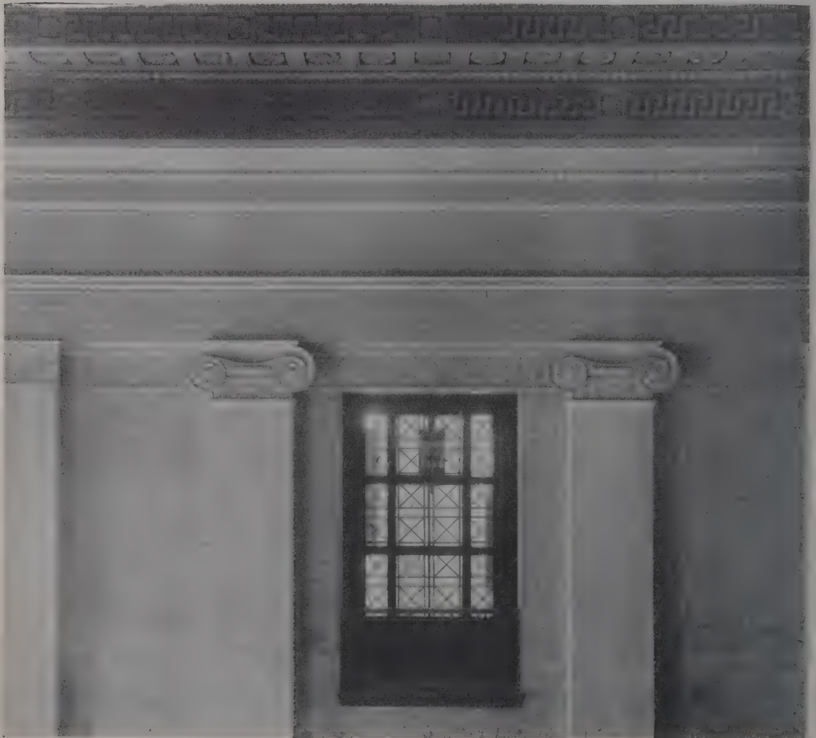
Wall Detail In Main Banking Room, Federal Reserve Bank, Birmingham, Ala.
