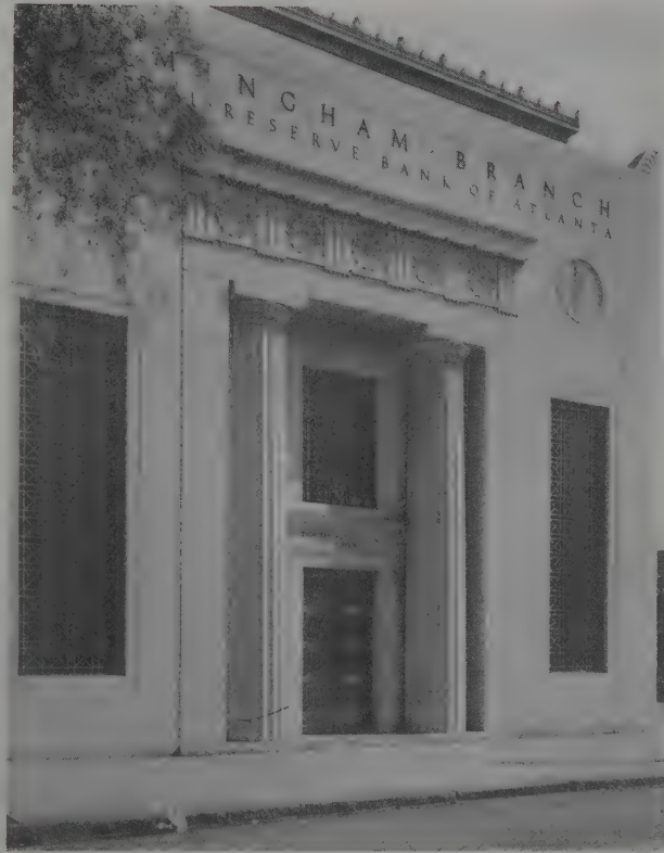
Entrance Detail, Federal Reserve Bank, Birmingham, Ala.
