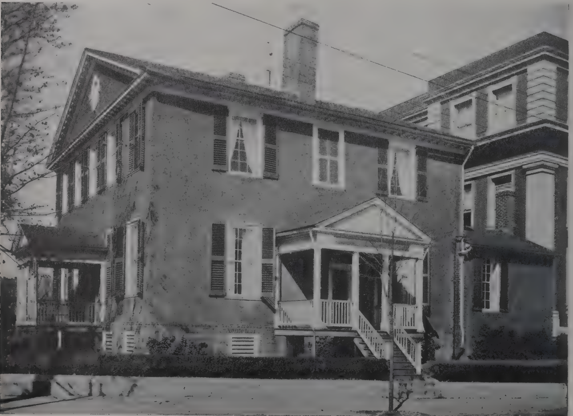
The Home of Chief Justice John Marshall, built 1810. The two entrance porticos are interesting.
