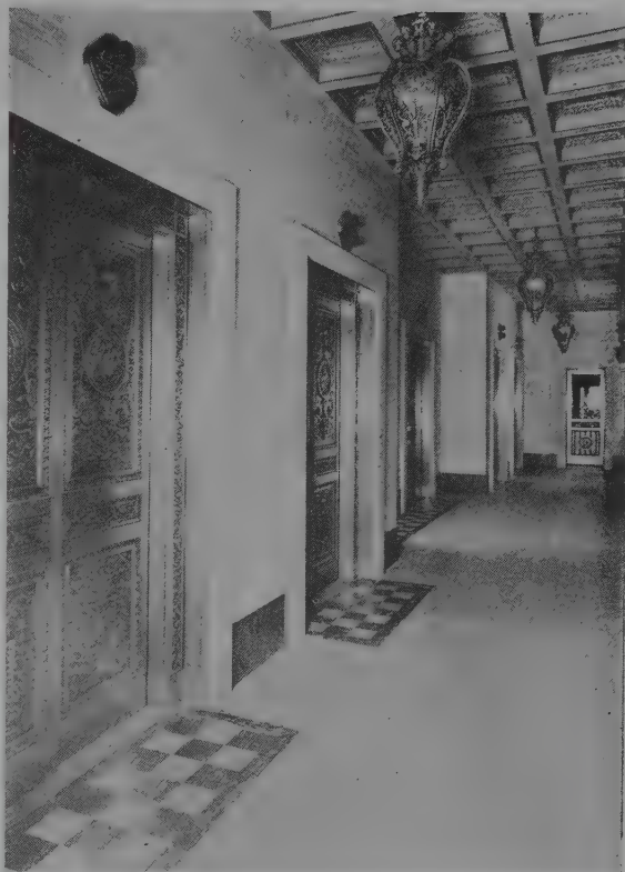
Six Signal Control Elevators with a Speed of Eight Hundred Feet Per Minute
