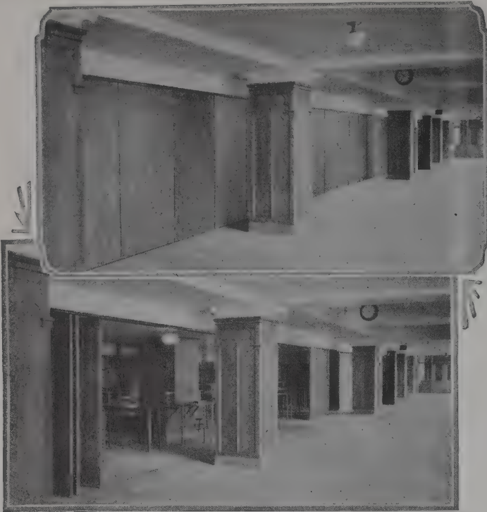
Weaver High School, Hartford, Conn. FRANK IRVING COOPER CORP., Architects A folding partition, 63 ft. in length, operating on Topping "Easyfold" Equipment, between the lunch room and cafeteria.
