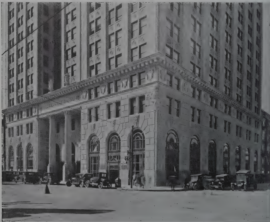
Architectural Treatment of Lower Portion of Building Showing Seven Foot Granite Base, Bedford Limestone Trim and Verde Antique Iron Window Frames
