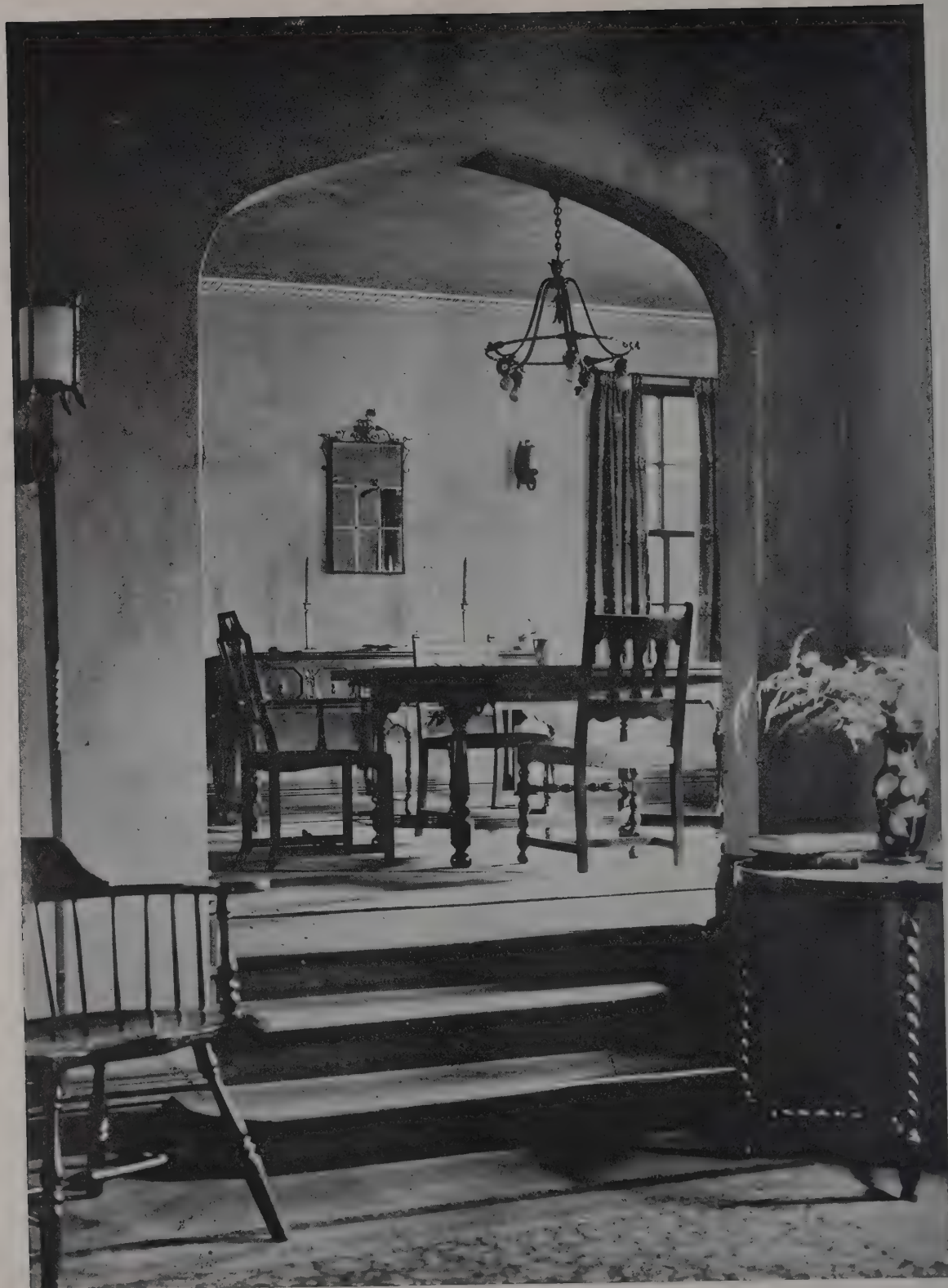
DINING ROOM DETAIL FROM LIVING ROOM HOUSE OF GEORGE MAHON, JR., MEMPHIS, TENN. GEORGE MAHON, JR., ARCHITECT
