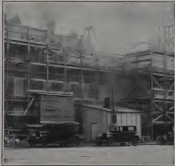
CAMBRIDGE, MASS. SISALKRAFT used for a windshield on staging. Note, too, that the field offices are covered with SISALKRAFT.
