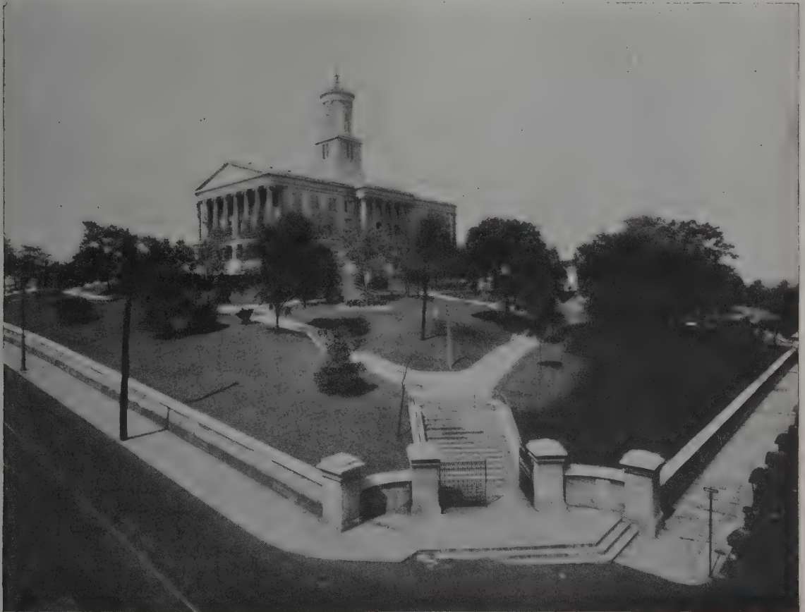
TENNESSEE STATE CAPITOL BUILDING, NASHVILLE, TENN. BUILT 1845, WILLIAM STRICKLAND, ARCHITECT.
