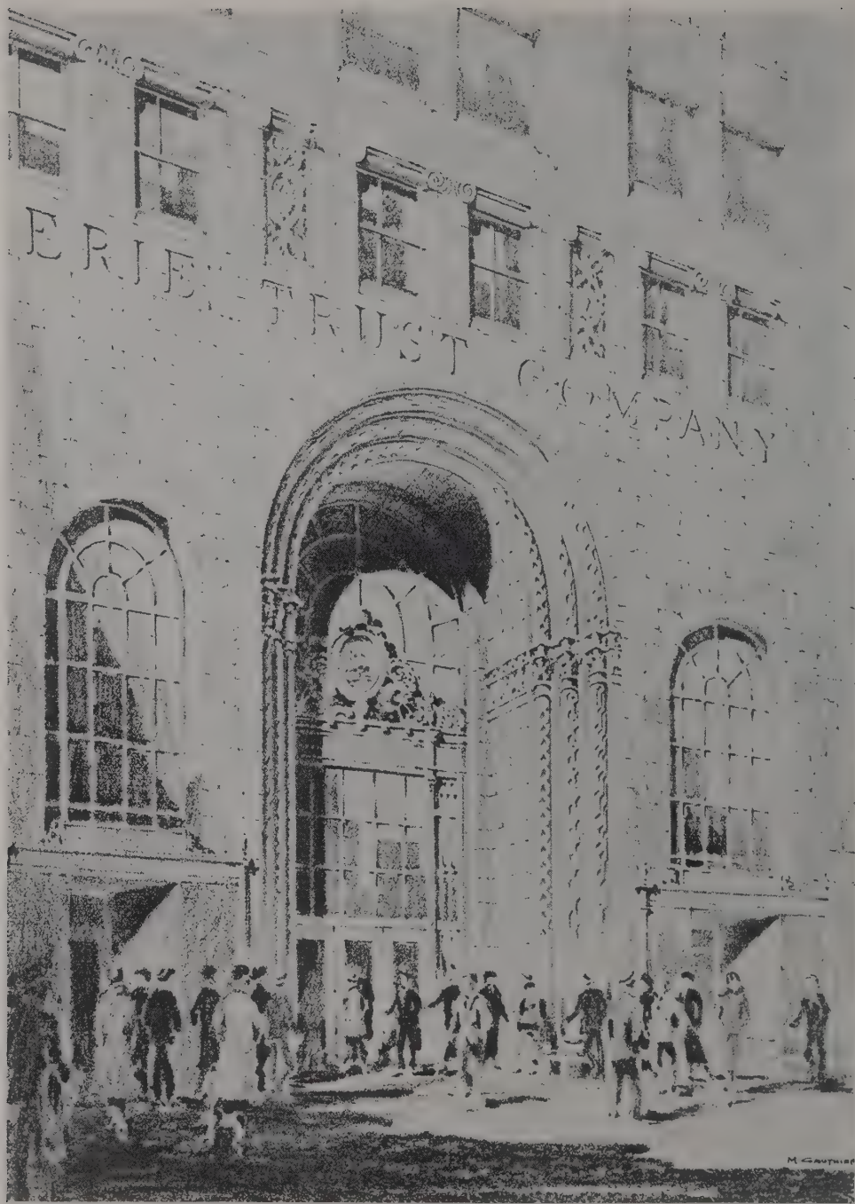
ENTRANCE DETAIL. ERIE TRUST COMPANY, ERIE, PA. DENNISON & HIRONS, ARCHITECTS.
