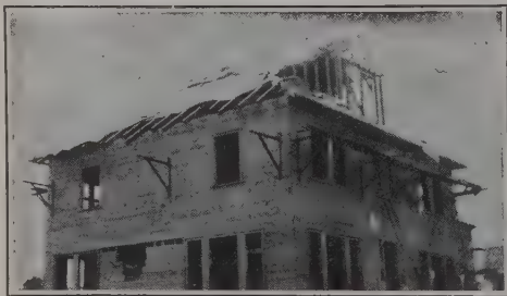
SISALKRAFT used for temporary roof to enable workmen to continue during a storm, and not hold up schedule.
