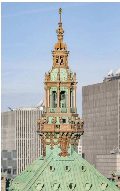
Thornton Tomasetti restored the Helmsley Building’s crowning cupola at the top of the pyramidal roof.
