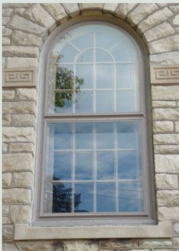
Exterior QUANTAPANELS with a custom color upgrade the energy efficiency of the Phoenixville Public Library's historic windows while protecting the exterior of the restored window unit.
