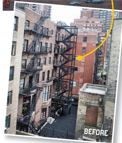
As part of the renovation, the unsightly fire escapes that obscured the façade were removed and a missing section of cornice was recreated.
