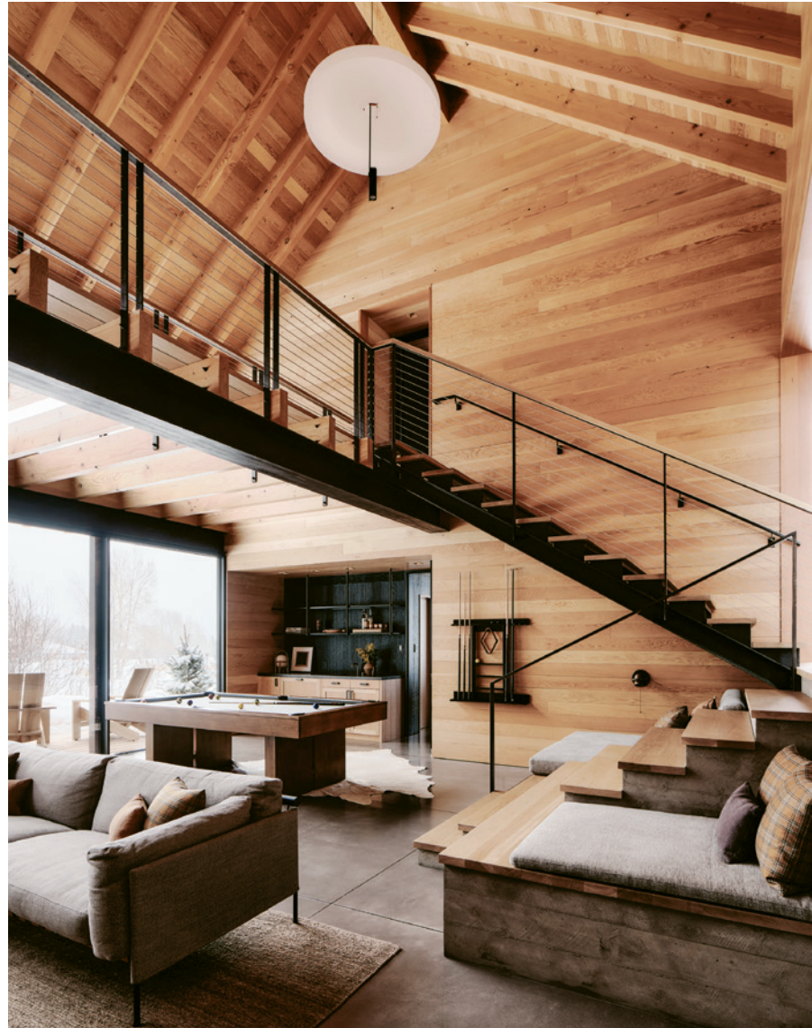
The playful kids' barn is entered at midlevel, left of the entry hall. A steel beam supports the catwalk's joists, which extend outside to cover a porch.
