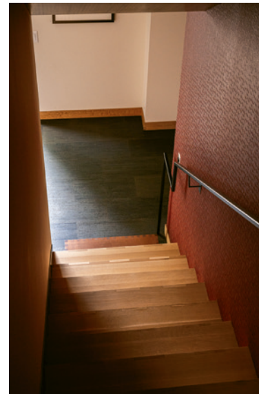
On the garage/guest volume, red woven vinyl fabric covers the stairwell walls, eliminating the need for trim. The floor in the connector is cork.
