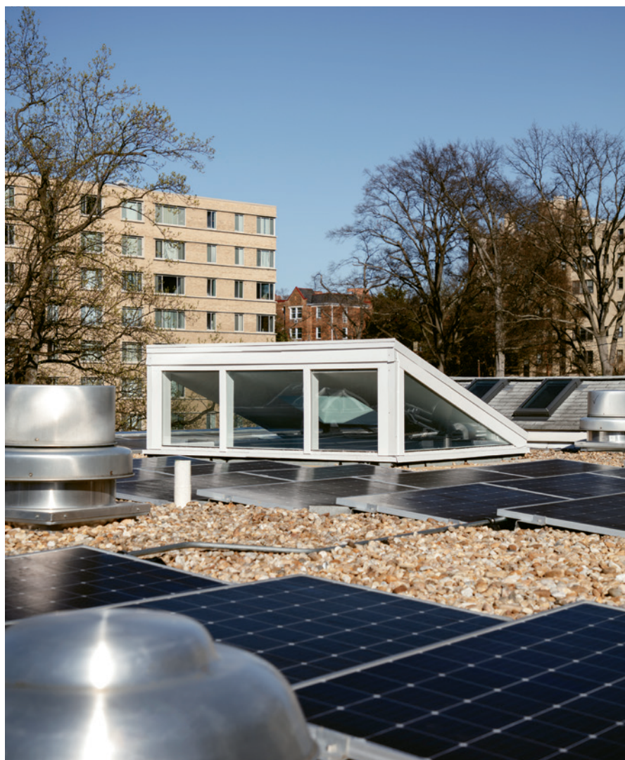
Built as an integrated skylight and window assembly, the apartment's single-slope roof structure stays out of view of the neighboring unit's skylights.
