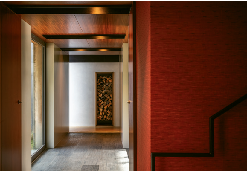
On the garage/guest volume, red woven vinyl fabric covers the stairwell walls, eliminating the need for trim. The floor in the connector is cork.
