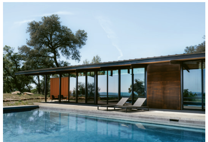
Stretching east-west, the bar-shaped living/dining/kitchen space opens south to the deep pool, which doubles as an emergency water source.
