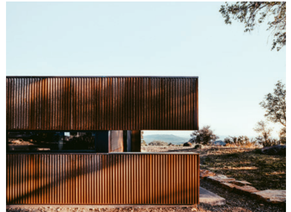
Hardy materials—corrugated steel, Napa stone, and concrete—offer high melting point resistance to future fires.
