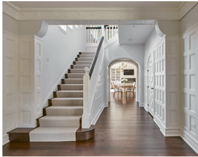
The architects had the foyer's dark wood paneling painted to brighten the interior, and reconfigured the stair for the modified height of the second-floor landing. Original stepped windows showcase their violet-tinted lites.
