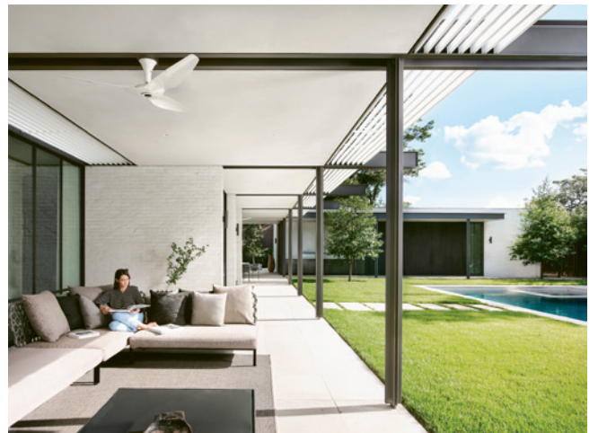
Wraparound steel trellises shade the west-facing rear of the house and tie together the main house, wing, and addition.
