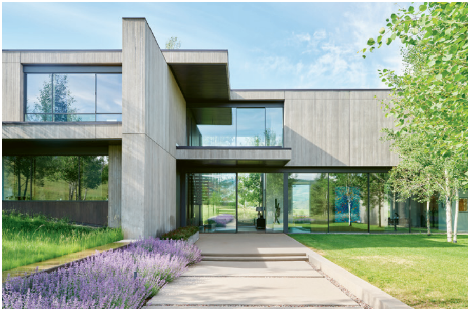
Mountain Modern: The solidness of vertical board-formed concrete contrasts with the transparent walls of glass at Mountain Modern. Dark stained oak adds warmth inside as well as to roof overhangs. A double-height wall hides the structure for the floating treads of the sculptural stair.
