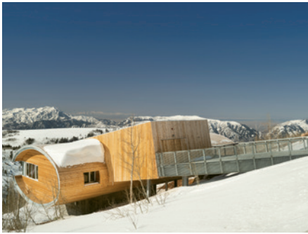
This page: House at 9,000 Feet by MacKay-Lyons Sweetapple is another stop on the home tour.
