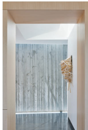
This page: Noise on this urban corner lot was intolerable until the firm deployed a board-formed concrete wall and designed a house around it.
