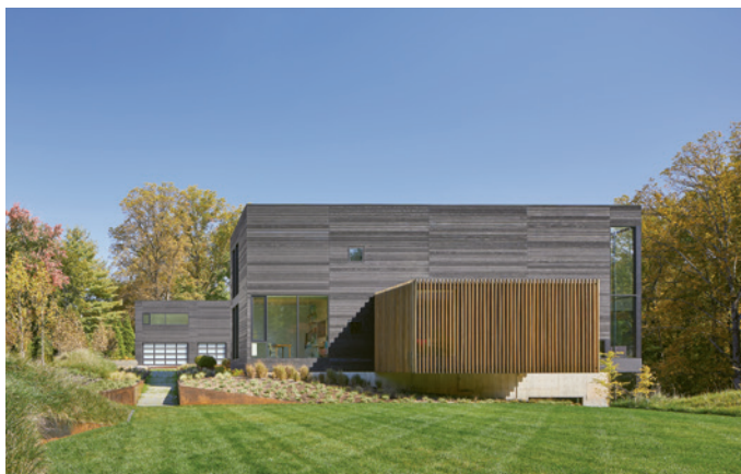
This page: The 18,000-square-foot house breaks down into a series of artful volumes to encompass the clients' hefty list of private and public spaces—including an Olympic-size indoor volleyball court and an indoor pool.
