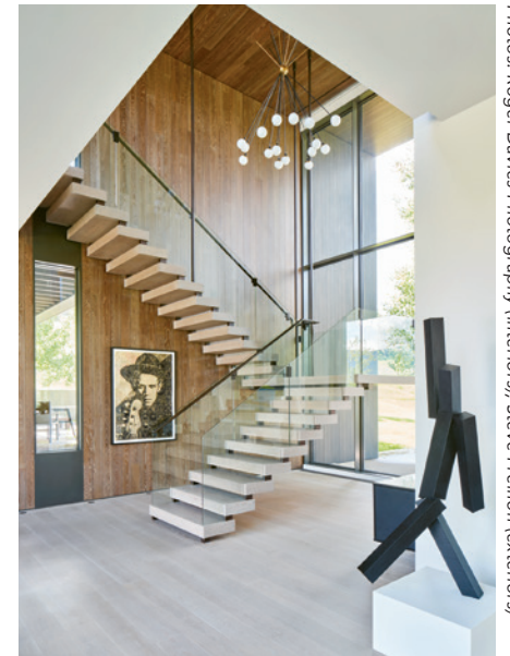
Mountain Modern: The solidness of vertical board-formed concrete contrasts with the transparent walls of glass at Mountain Modern. Dark stained oak adds warmth inside as well as to roof overhangs. A double-height wall hides the structure for the floating treads of the sculptural stair.
