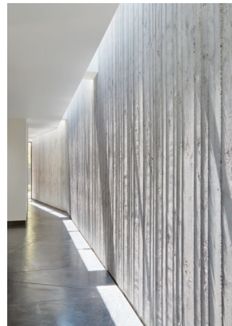
This page: Noise on this urban corner lot was intolerable until the firm deployed a board-formed concrete wall and designed a house around it.
