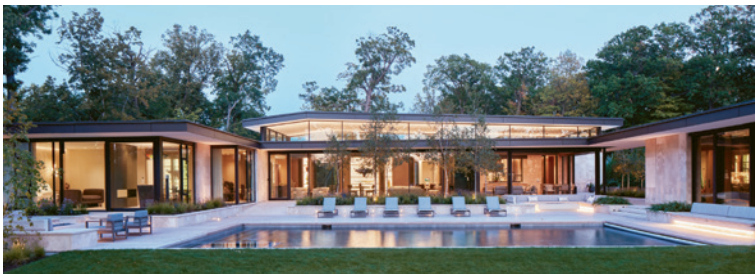
Midwest Sanctuary: Ramon Gray limestone clads the summer home Midwest Sanctuary while hand-carved niches into the stone add a personal touch. The house wraps around the courtyard and makes extensive use of glass to fulfill the owner’s wish for uninterrupted views of the pool terrace and neighboring golf course.
