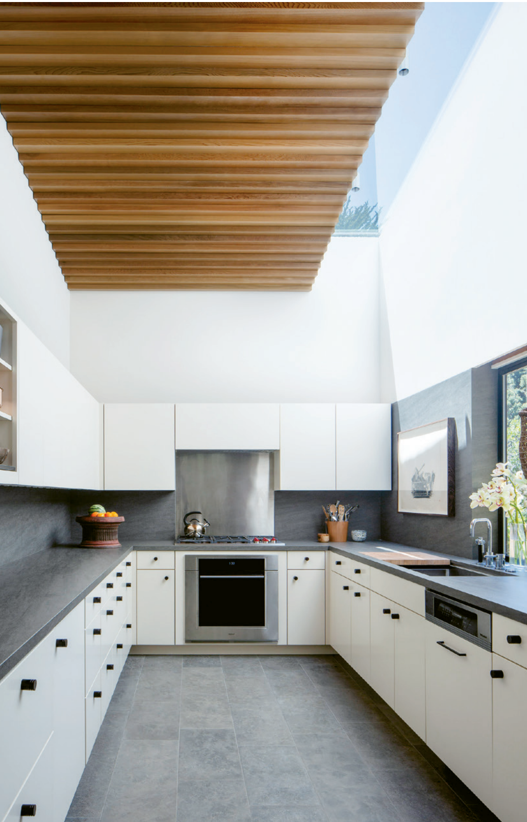
Cedar shiplap ceilings nod to the material of choice at Sea Ranch. In the kitchen, they stop just short of a skylight. Neolith counters and dark limestone floors confer the durability a family compound requires.
